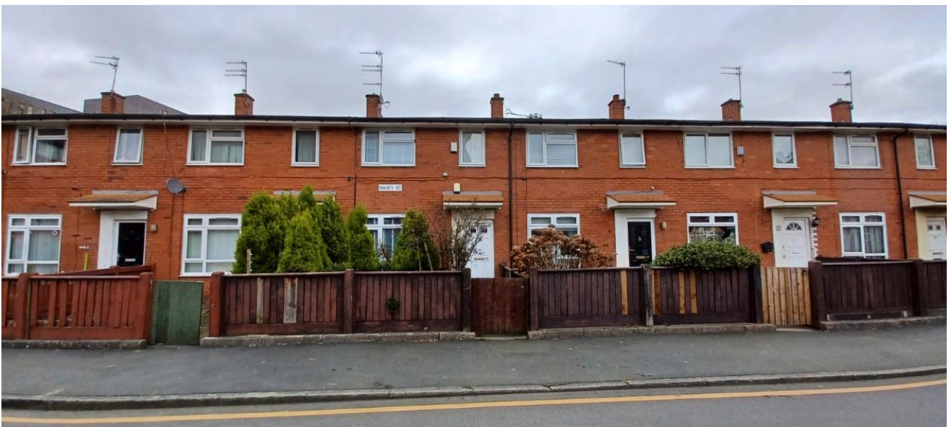
Figure 1. Principal elevation of No.33 Nancy Street.
