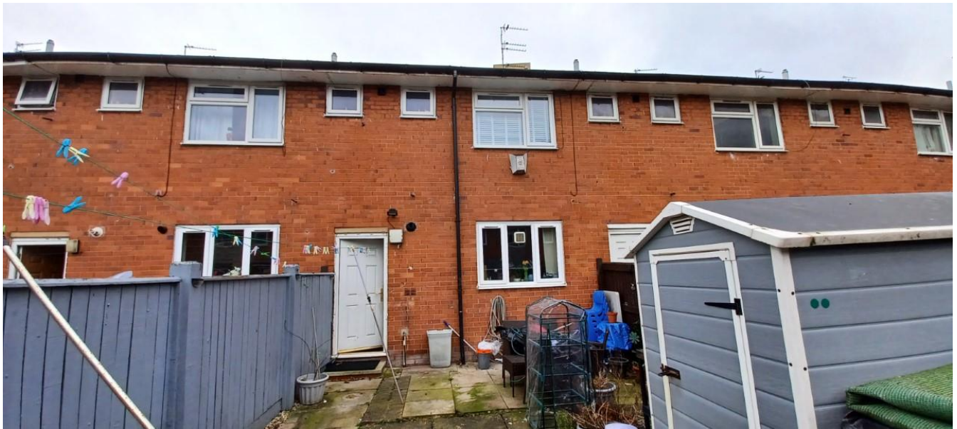
Figure 2. Rear elevation of No.33 Nancy Street.
