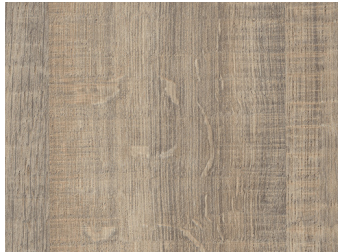
Stairs Floor Finish Existing floor to be cleaned sanded and stained.
