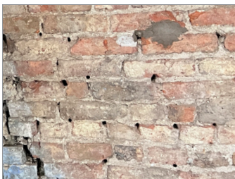
Wall Finish Retain Exposed Brick where possible.
