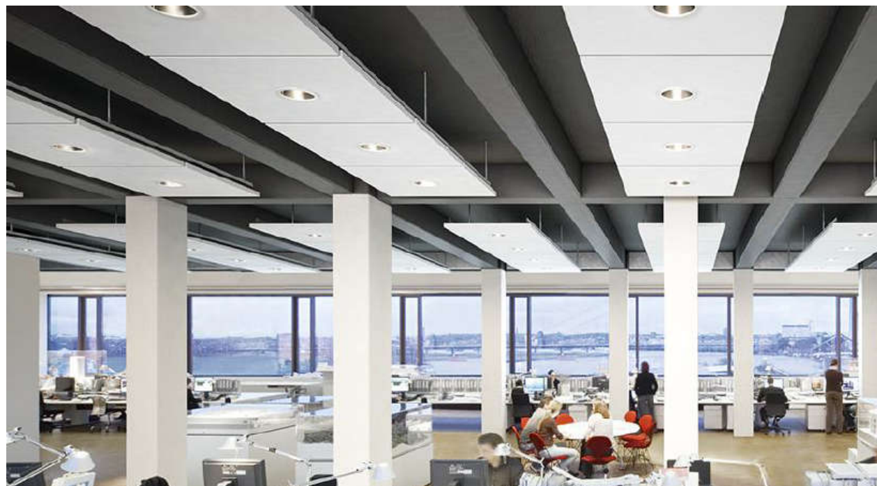
Figure 6.2: Suspended Absorptive Raft Panels with Recessed Light Fittings
