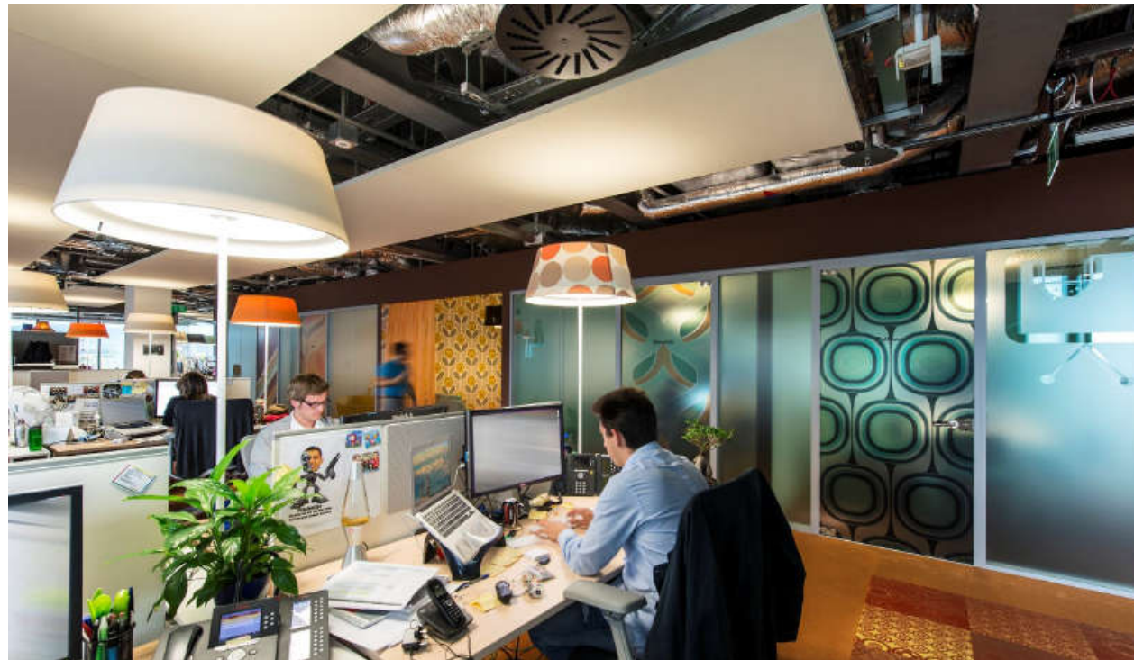
Figure 6.2: Suspended Absorptive Raft Panels with Recessed Light Fittings
