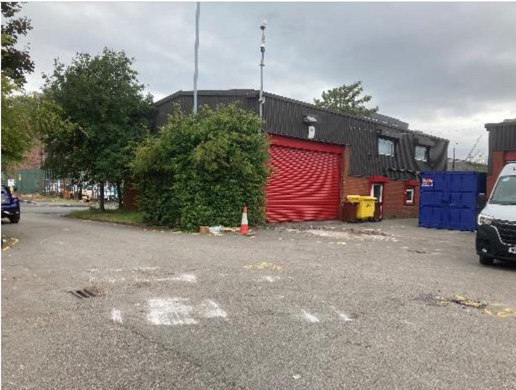
PLATE 2 VIEW OF SITE FACING WEST
