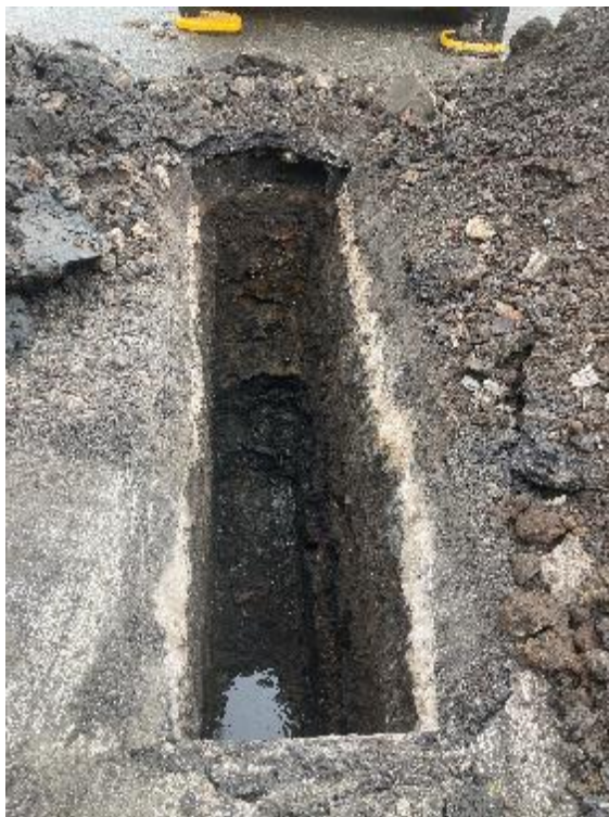
PLATE 4 TP102 ARISINGS AND EXCAVATION
