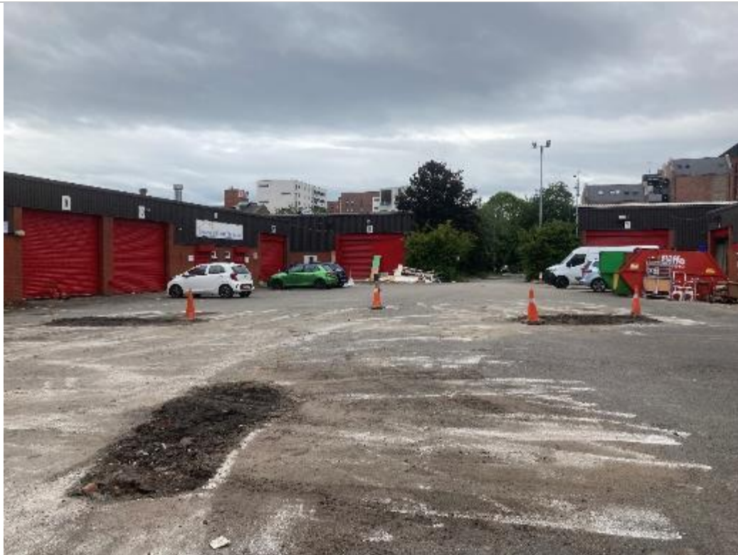
PLATE 3 VIEW OF SITE FACING WEST
