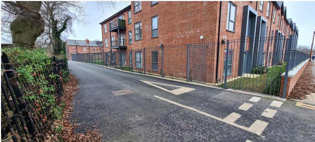
Figure 4: Existing vehicular access to Church with northern site boundary on left.
