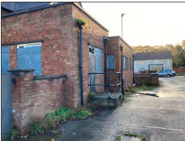
General view to south east along side of the main building
