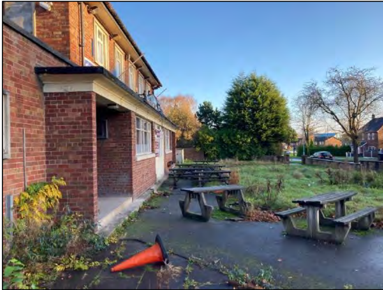
View along front of building
