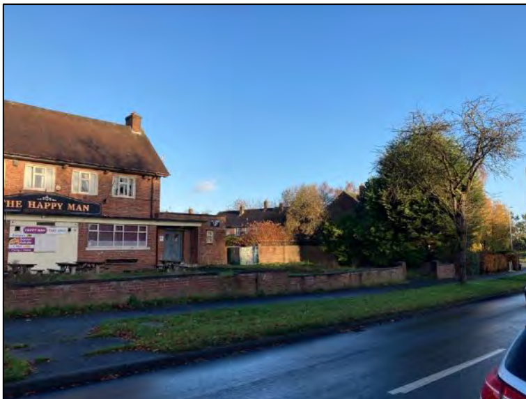
General view to north from Portway
