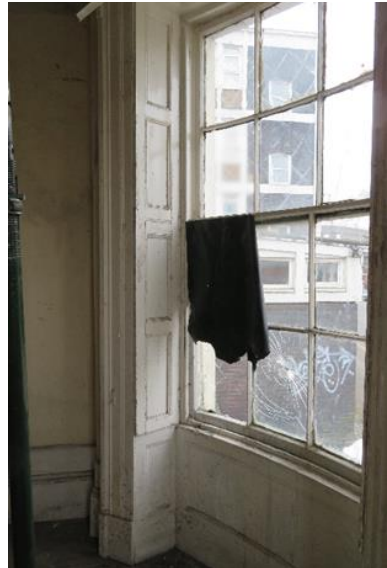
Left: Early deep cornice on upper ground floor. Centre: Plinth, architraves and panelled casings to upper floor windows. Right: Bay sash window and shutters on the upper ground floor.
