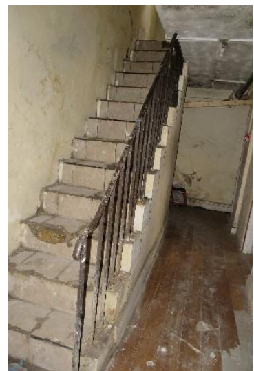
Left: Basement corridor with low ceilings and plain walls and floor. Right: Simple square section balustrades and wrought iron handrail to basement stairs. [stone treads/risers?]
