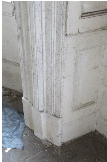
Left: Early deep cornice on upper ground floor. Centre: Plinth, architraves and panelled casings to upper floor windows. Right: Bay sash window and shutters on the upper ground floor.
