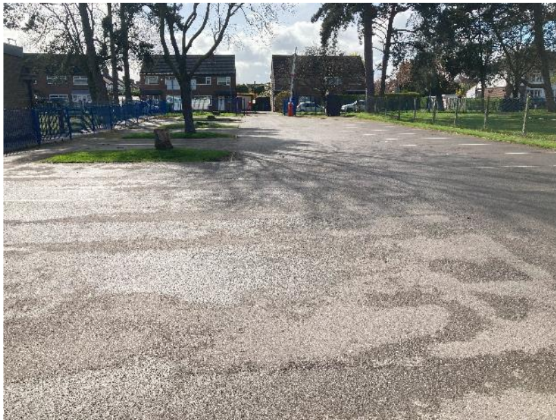
PLATE 1 SHOWING AREA OF HARDSTANDING
