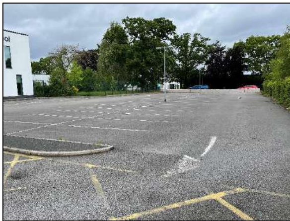
Figure 17: Areas of tarmac parking and access.
