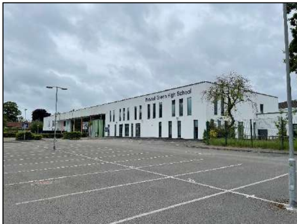
Figure 19: Looking at the building from the east.
