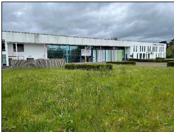
Figure 3: Looking north at the school buildings.
