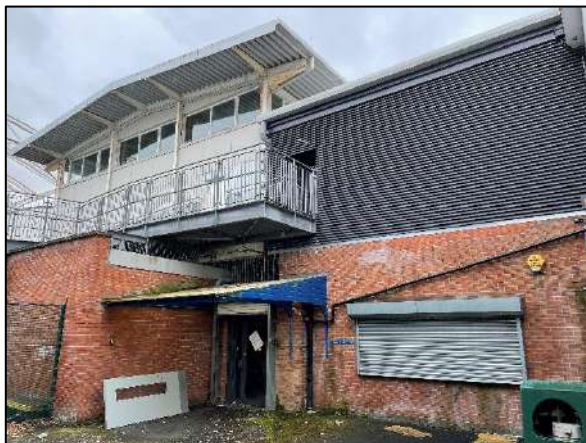
Figure 33: The varied construction of the building.
