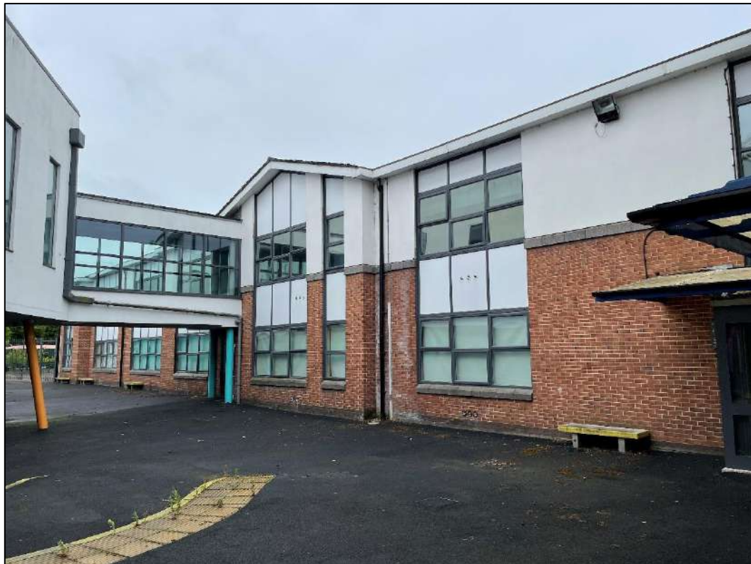
Figure 32: Building 1 viewed from an internal courtyard between Buildings 1 and 2.
