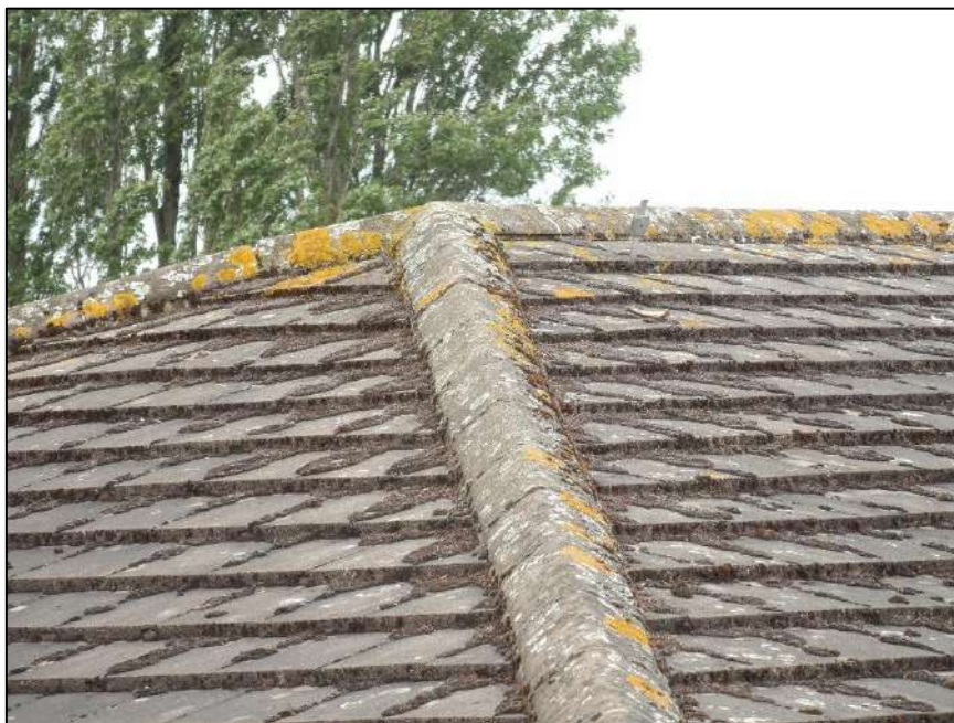
Figure 39: The tight fitting cement tiles and sealed ridge and hip tiles.
