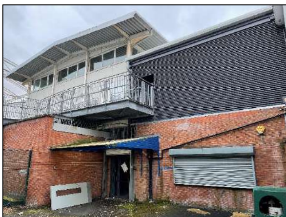
Figure 40: The large area of louvred wall.
