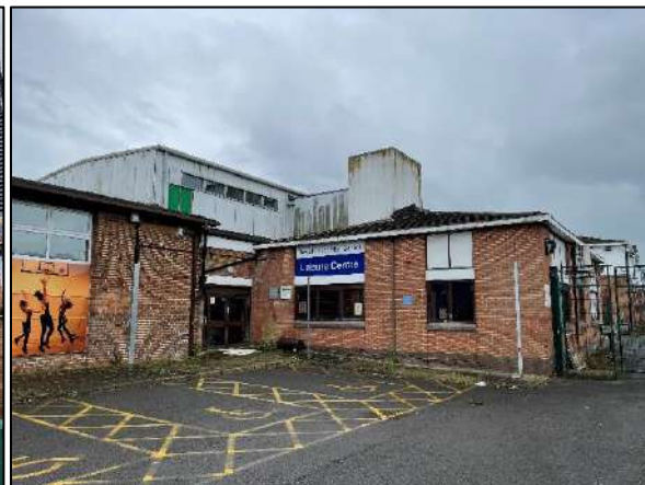
Figure 34: The western elevation of the building.
