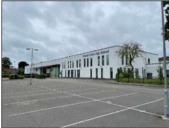
Figure 42: The southeast elevation of the building.
