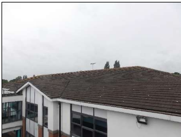
Figure 35: One of the hipped cement tiled roofs.
