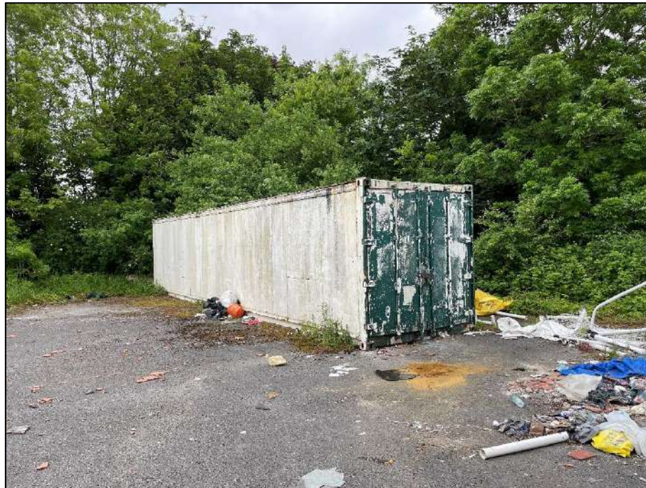
Figure 21: The cargo container located in the parking area.
