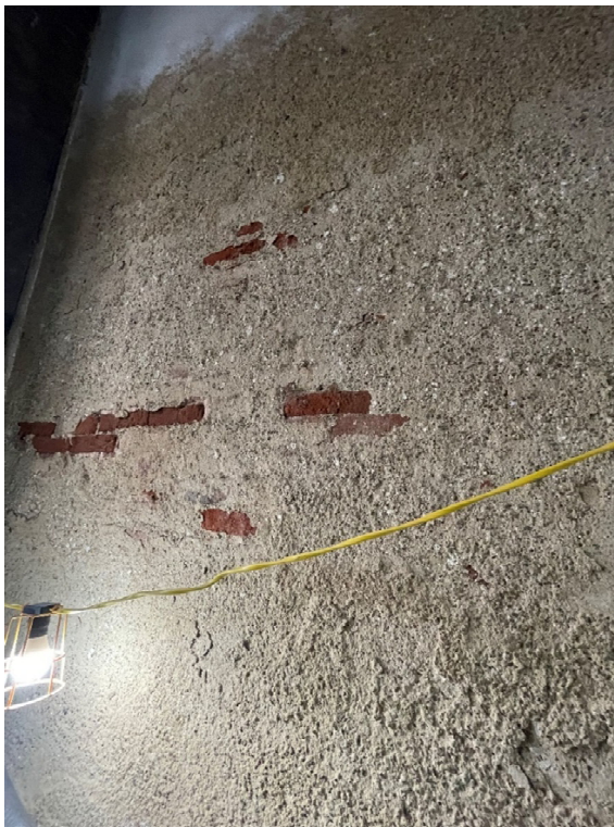
Figure 2 Defective plaster
