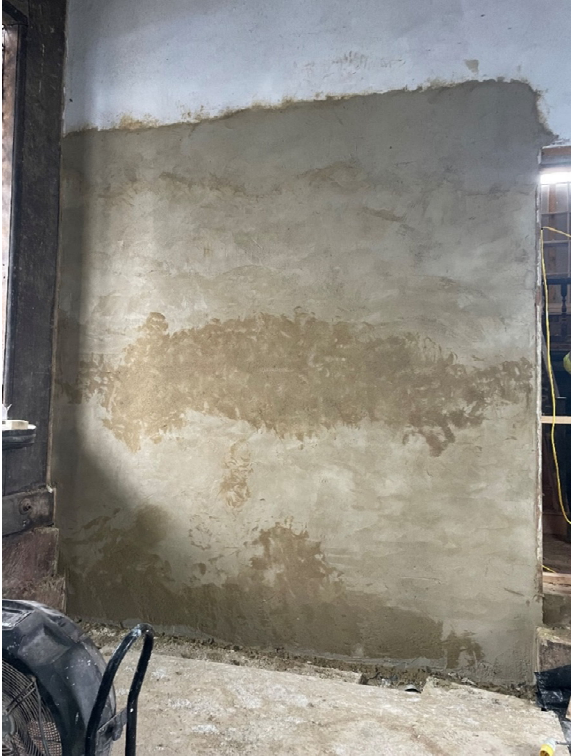
Figure 4 Sample of plaster finish
