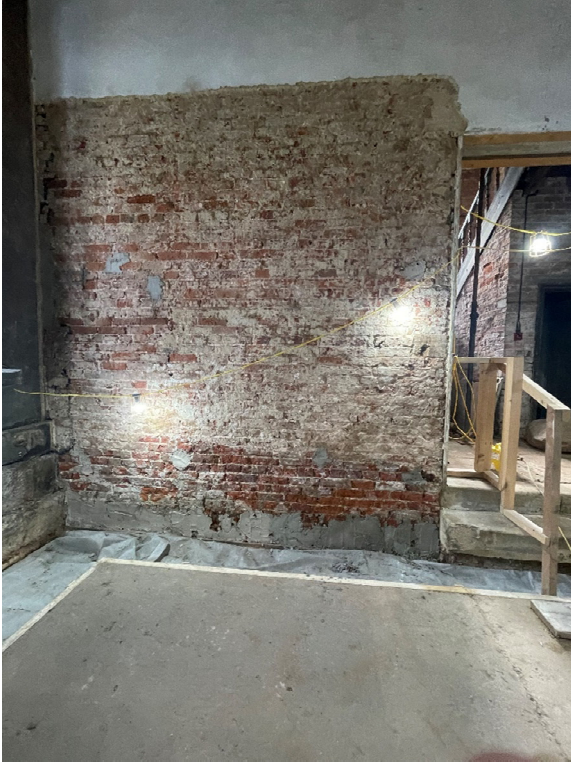
Figure 3 Defective plaster removed, and brickwork dubbed out
