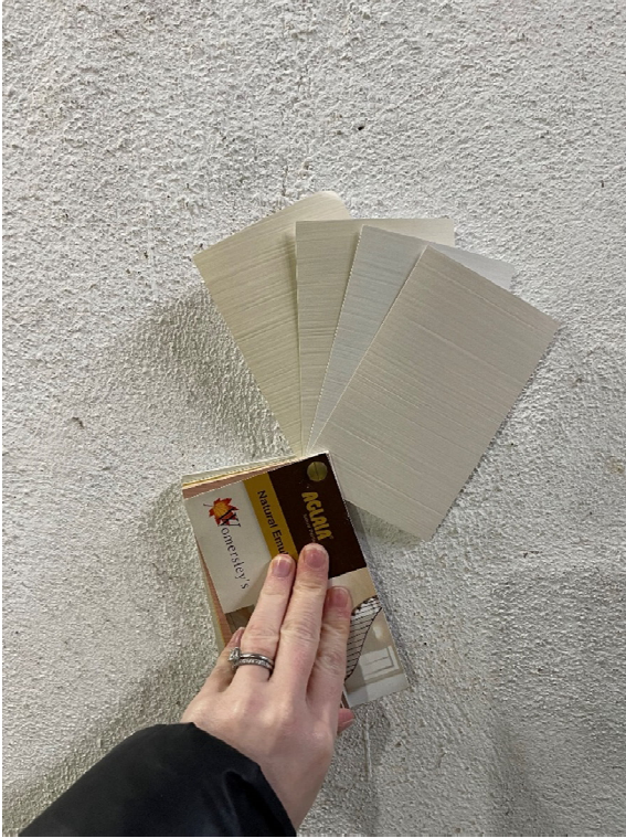
Figure 5 Colour match to existing painted finish
