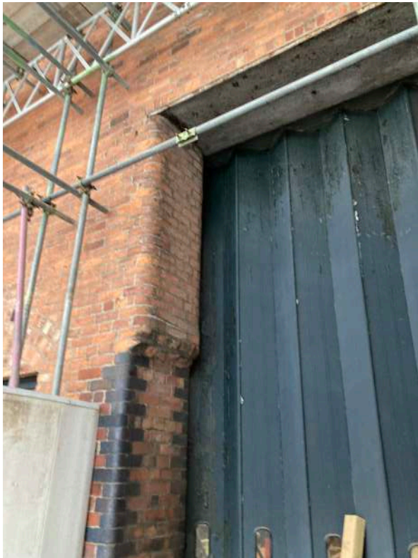
Corbelled brickwork at the top of the opening of the small aperture
