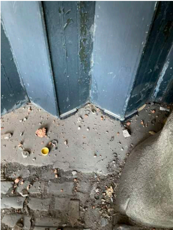
Full carriage stone within the depth of the reveal
