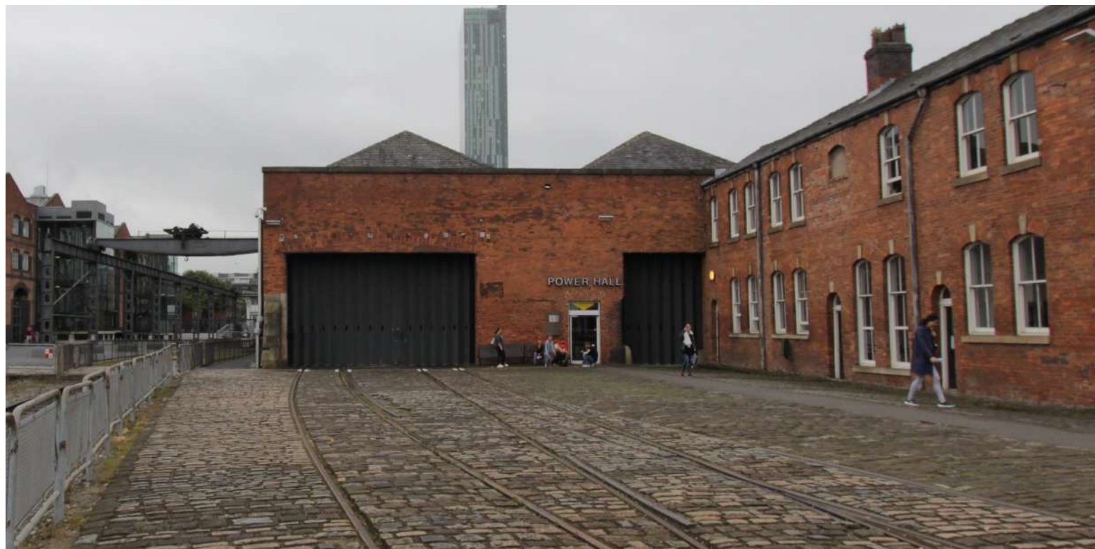
The west façade prior to construction work with modern fully glazed single door set
