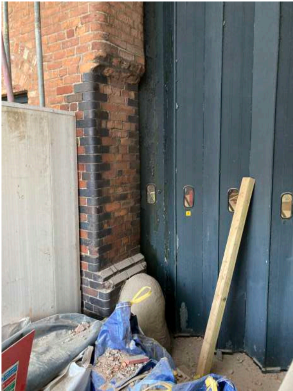
Corbelled brickwork at the base of the small aperture and carriage stone
