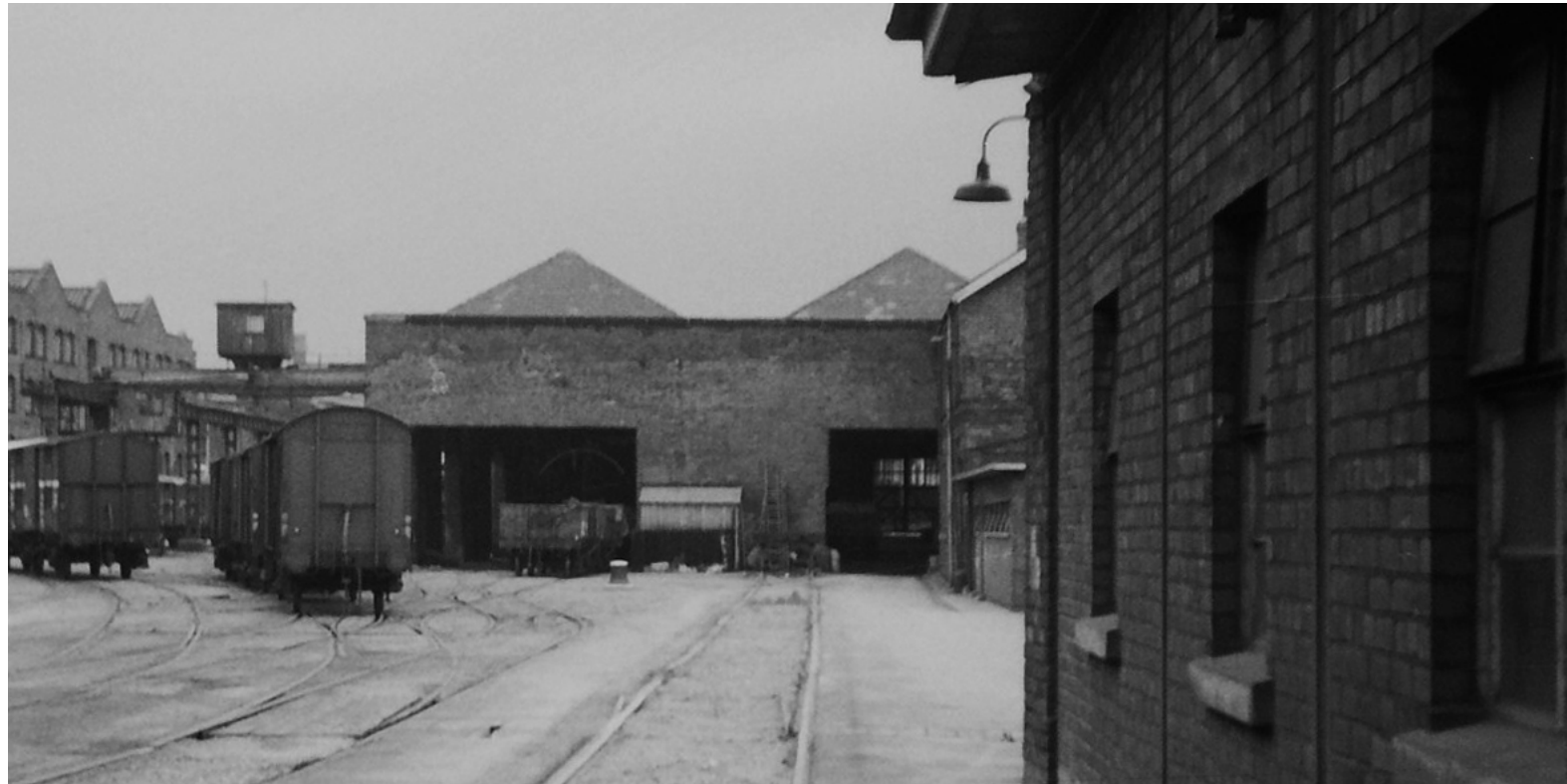
The west façade in 1973 without the modern fully glazed single door set
