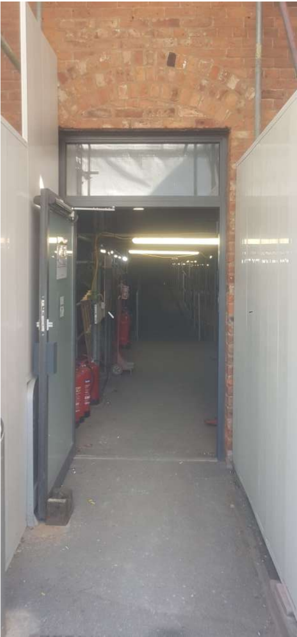
Non-original modern glazed single door set, and existing fire escape
