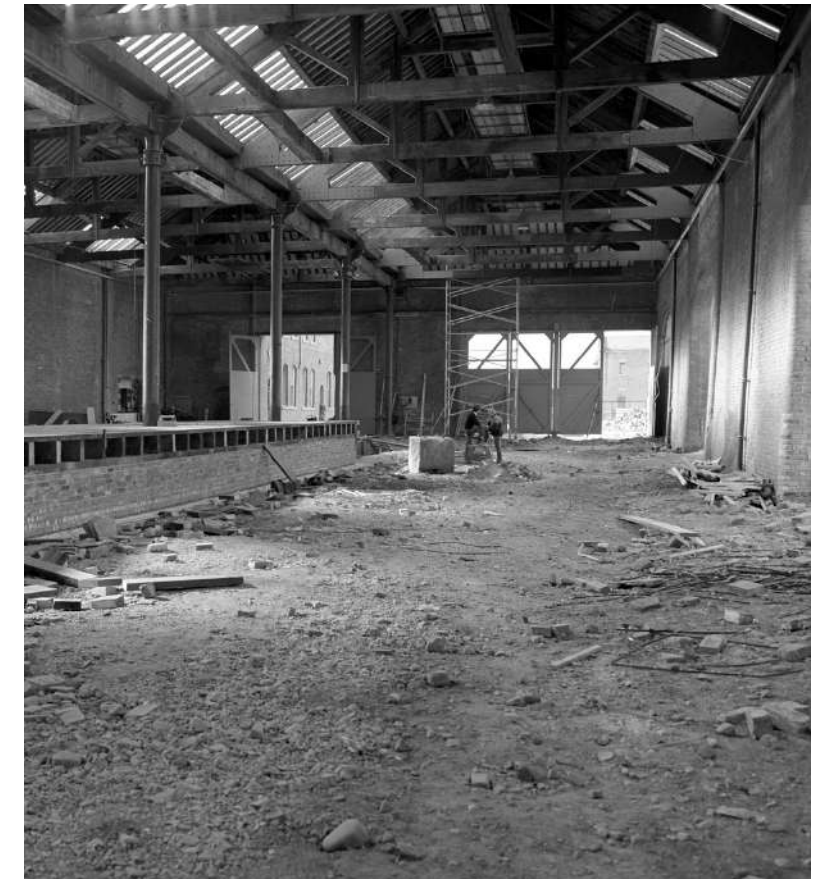
View of the Shipping Shed during restoration, 1981 (SIM)
