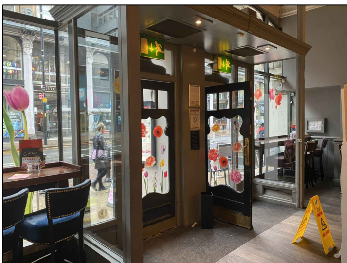
IMAGE REF 3: EXISTING ENTRANCE LOBBY
