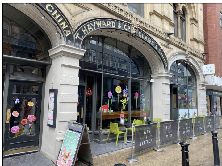
IMAGE REF 2: EXISTING SHOPFRONT
