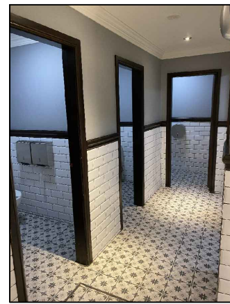
IMAGE REF 18: EXISTING LADIES CUBICLES
