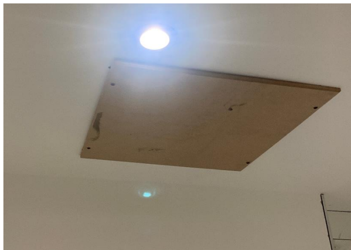
Fig 4: Low Energy LED Lighting
