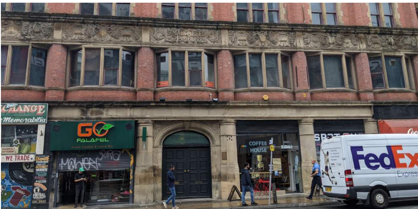
Photograph of Ground Floor Units on Newton Street
