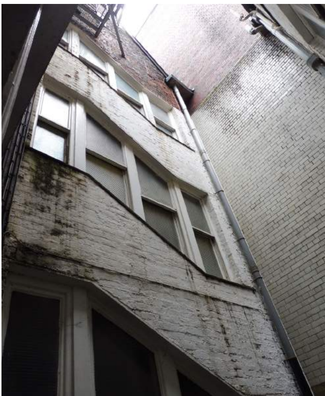
Photograph of Lightwell
