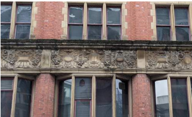
Photograph of Exterior Detailing
