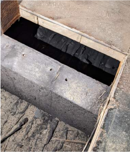
Photograph of Existing Floor Build up
