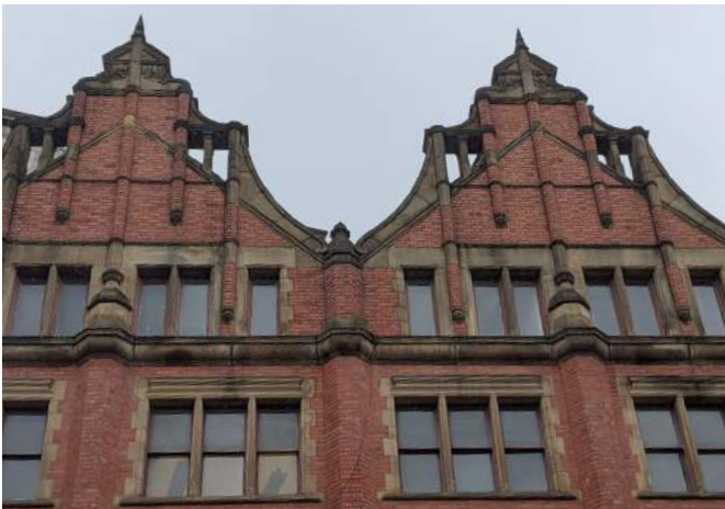
Photograph of Exterior- Upper Floors
