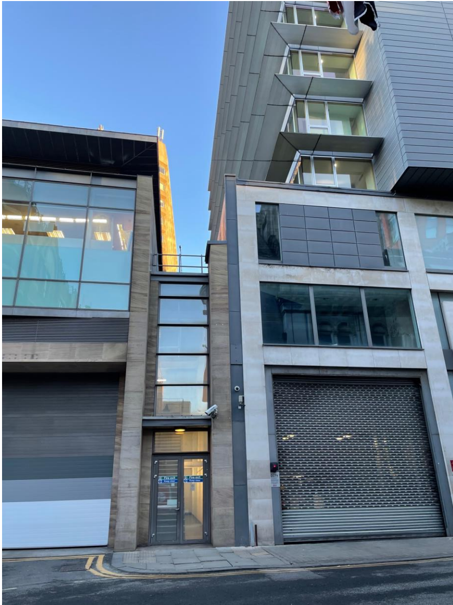
Photograph 4: View from Norfolk Street - distance approx. 30m (No line of sight to proposed new equipment from this viewpoint)
