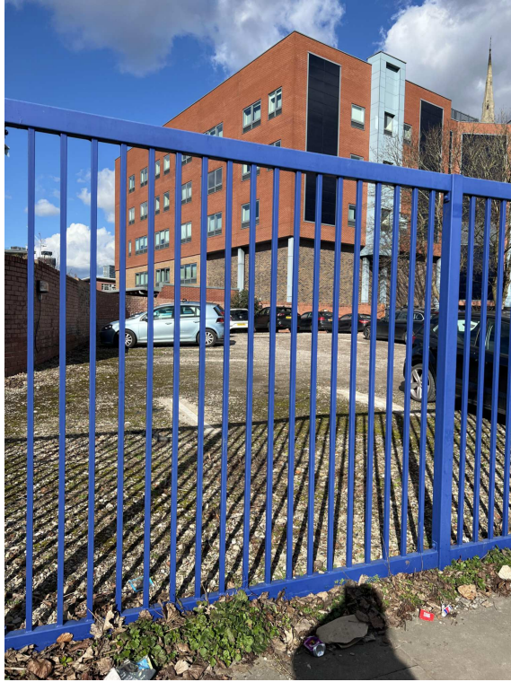
2 - View of existing fence from footpath towards E&K building.
