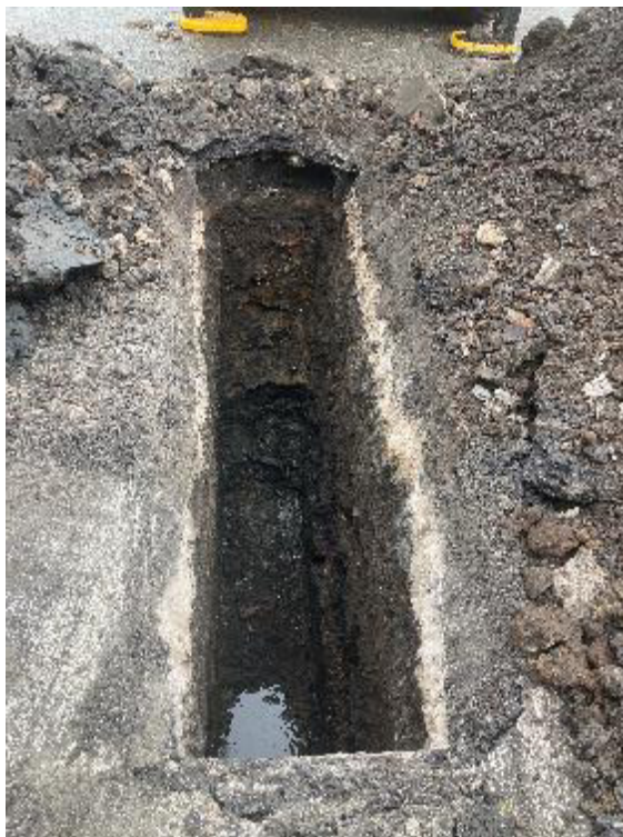
PLATE 4 TP102 ARISINGS AND EXCAVATION
