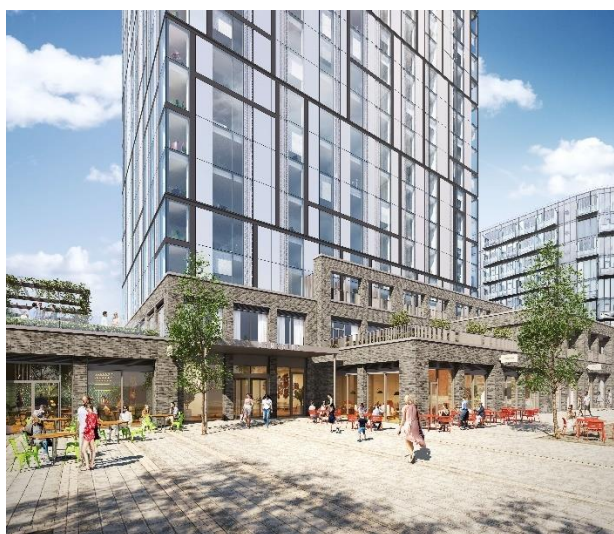
Figure 15: Bankside at Colliers Yard CGI
