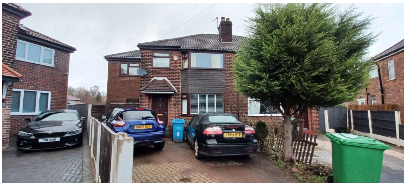
Figure 1. Photograph of the principal elevation of No.8 Moresby Drive.
