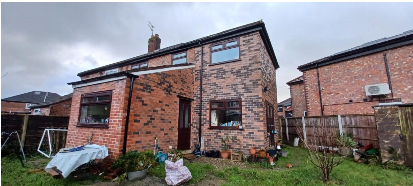
Figure 2. Photograph of the existing single-storey rear and two-storey side extensions present at the property.
