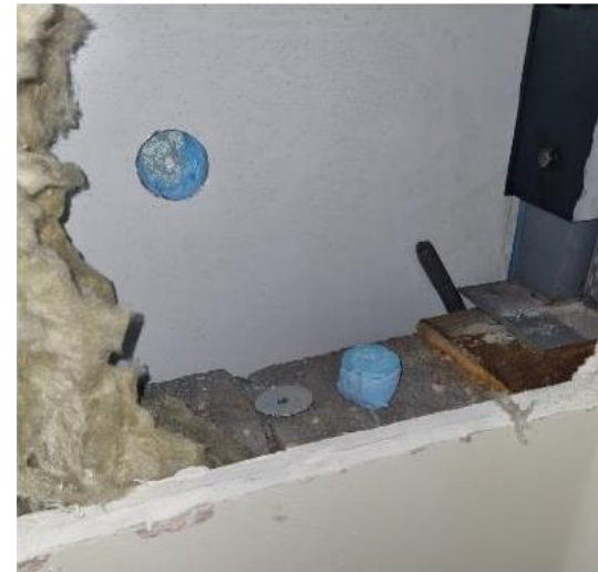
Figure 15: Core sample of spandrel panels Image from the Global Report Above
