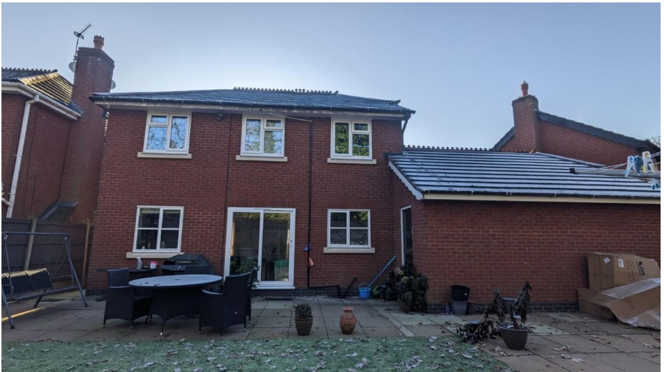
Figure 2. Photograph of the rear elevation of No.67 Bronington Close.
