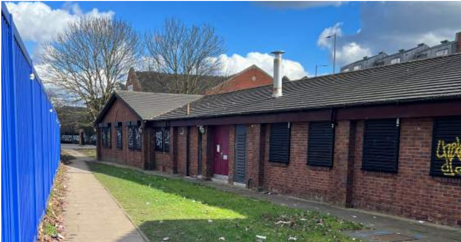
View along Existing Footpath in Centre of Site looking East
