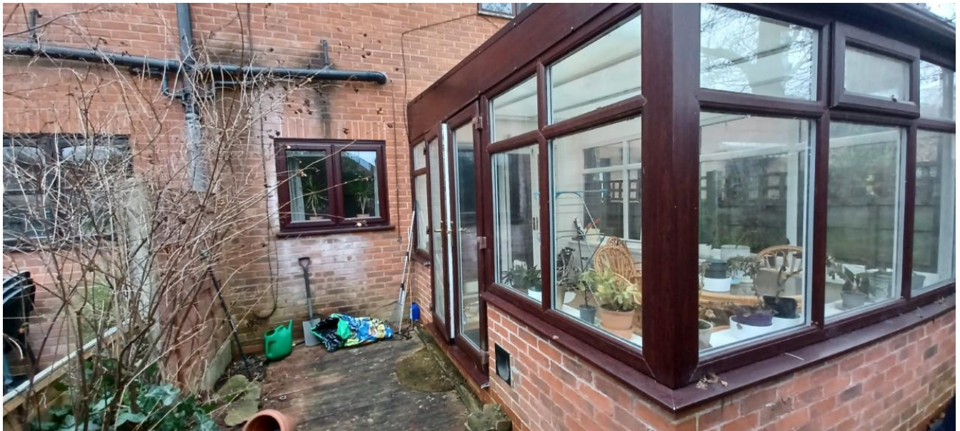
Figure 2. Existing conservatory located to the rear.
