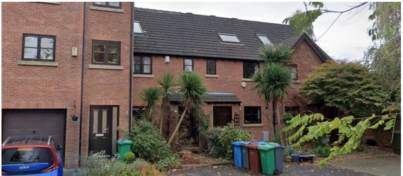
Figure 1. Principal elevation of No.10 Dovecote Mews, as seen on Google Maps.
