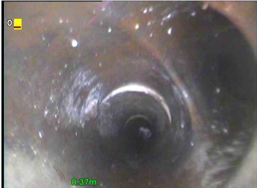
, 00:00:20, 0.37 m Junction at 2 o'clock, diameter: 100mm
