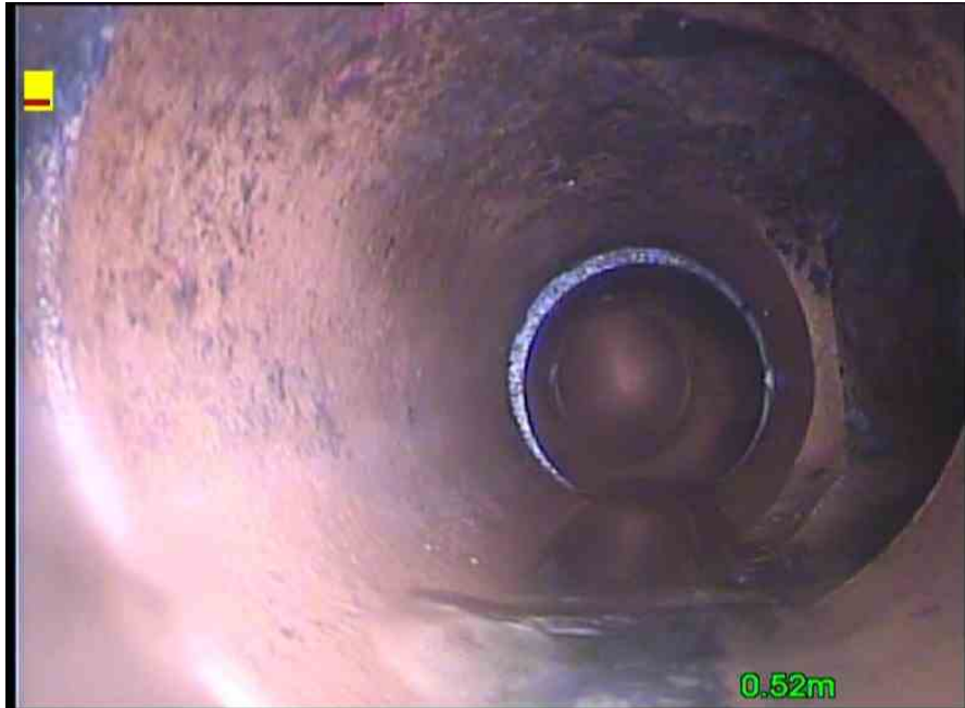
, 00:00:10, 0.52 m Junction at 3 o'clock, diameter: 100mm
