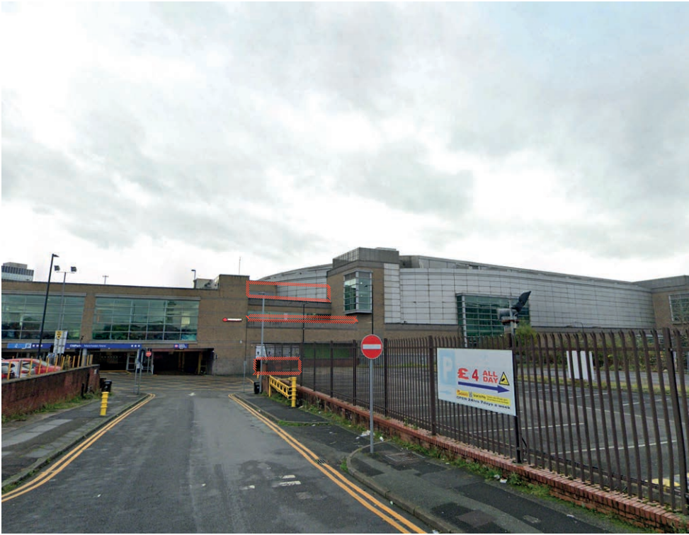
Existing view from Dutton Street looking towards the Trinity Tunnel
