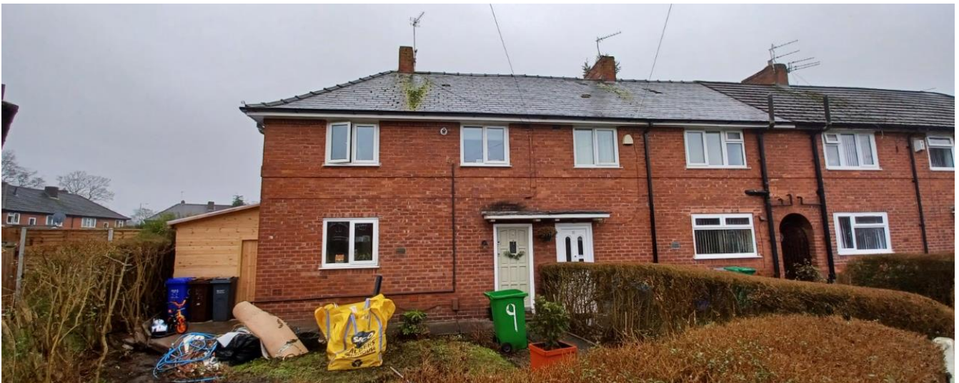
Figure 1. Photograph of the principal elevation of No.9 Pingot Avenue.
