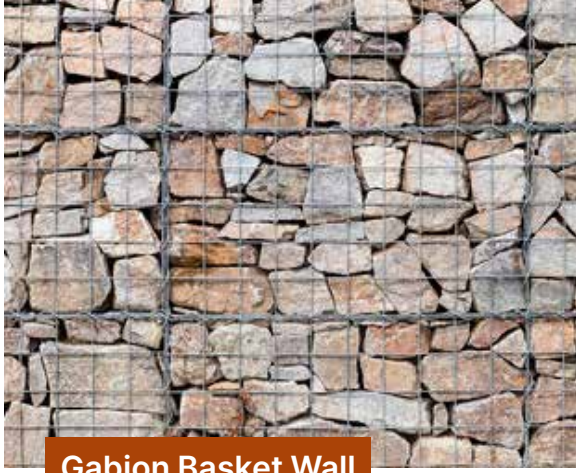
Gabion Basket Wall
