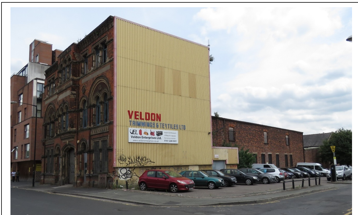
Figure 2 – Looking south-east towards the principal front (left) and side elevation from Laystall Street.
