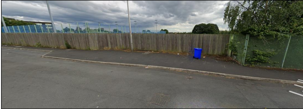
Figure 4.3 - Photograph showing existing timber and metal mesh fencing
