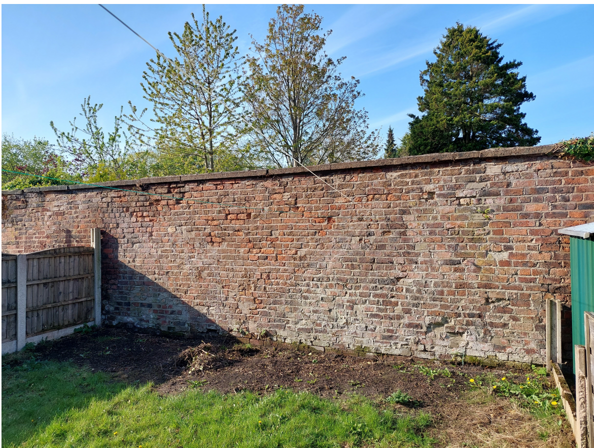
Existing rear boundary wall
