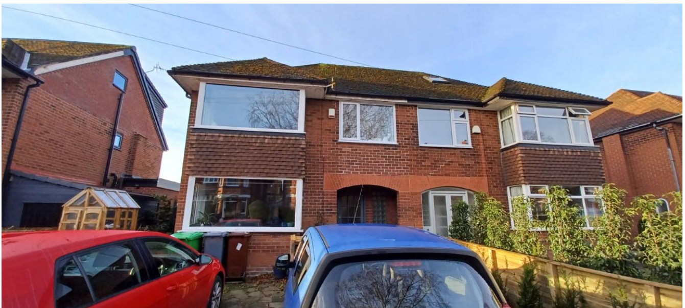
Figure 1. Photograph of the principal elevation of No.16 Moorland Road.
