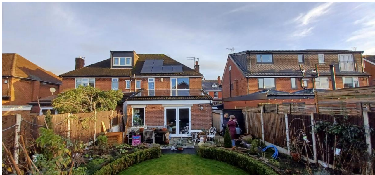
Figure 2. Photograph of the rear elevation of the property, depicting the existing rear extension.
