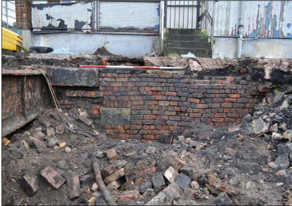
Plate 19. Northwest face of wall 402, facing southeast
