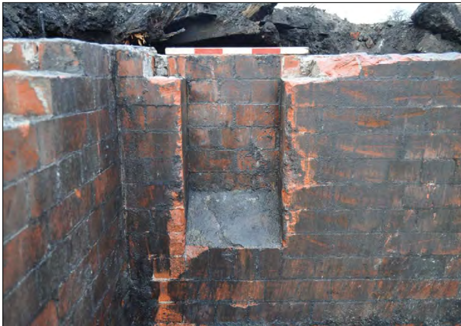
Plate 16. Example of alcove in southeast interior face of wall 317, facing northeast
