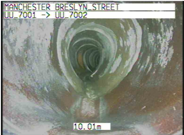
UU_7001X_204cf936-b952-4a7a-ba41-949c8656d6f7_20220914_112307_282.jpg, 00:01:30, 10.01 m Shape changes to egg-shaped, new size(s), 300mm high, 150mm wide
