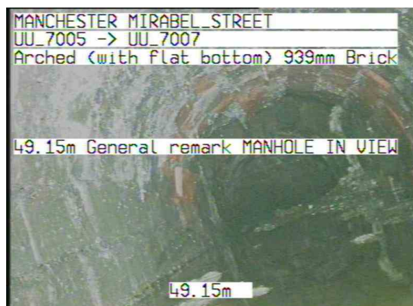
UU_7005X_b2acda02-03ab-403f-9812-f903a72371f7_20220914_103157_784.jpg, 00:08:03, 49.15 m General remark, MANHOLE IN VIEW
