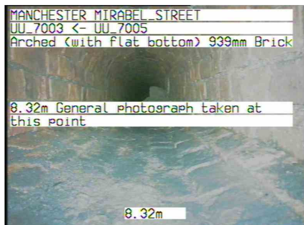
UU_7003X_4a89acd2-31d0-4228-878b-4576d76e746e_20220914_104958_559.jpg, 00:01:42, 8.32 m General photograph taken at this point
