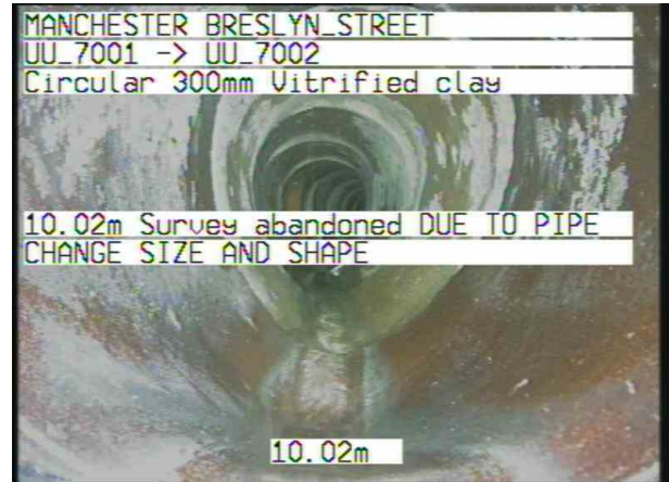
UU_7001X_f4b55c27-c717-4821-b113-a1d981659c8d_20220914_112323_193.jpg, 00:01:37, 10.01 m Survey abandoned, DUE TO PIPE CHANGE SIZE AND SHAPE
