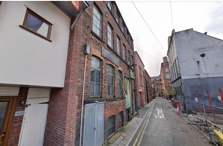
3. View along Bank Street with site on right
