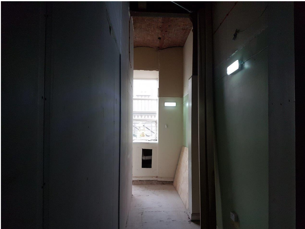
Image 006: Fire Escape Corridor
