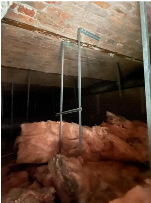
Image 012: Above ground floor suspended ceiling
