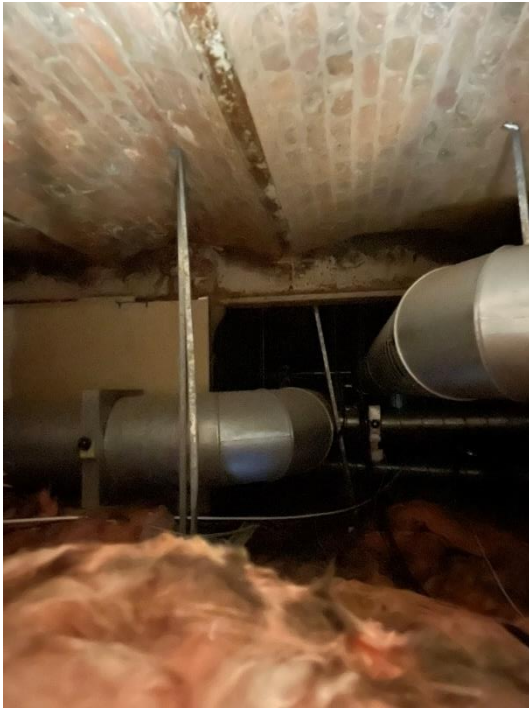
Image 010: Above ground floor suspended ceiling
