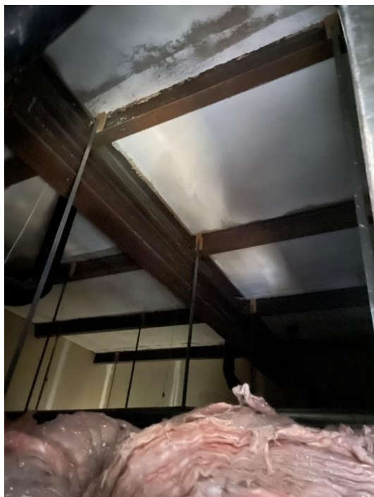
Image 017: Ground floor office typical interior
