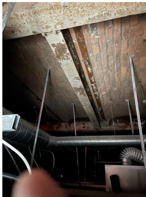
Image 009: Above ground floor suspended ceiling
