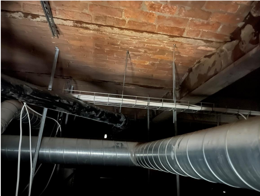
Image 007: Above ground floor suspended ceiling
