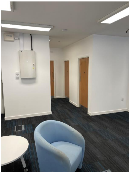
Image 016: Ground floor office typical interior
