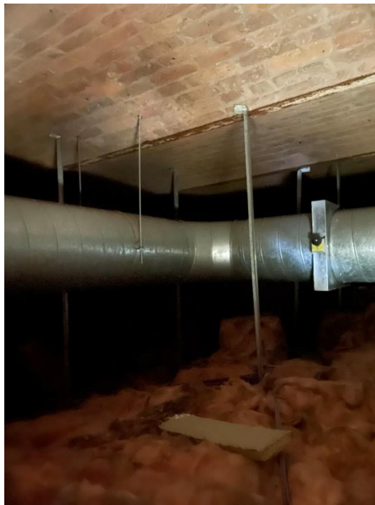
Image 011: Above ground floor suspended ceiling
