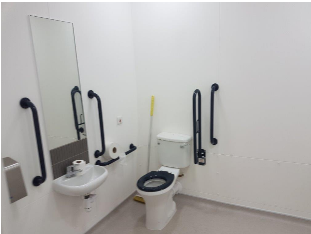
Image 021: Ground floor office toilet
