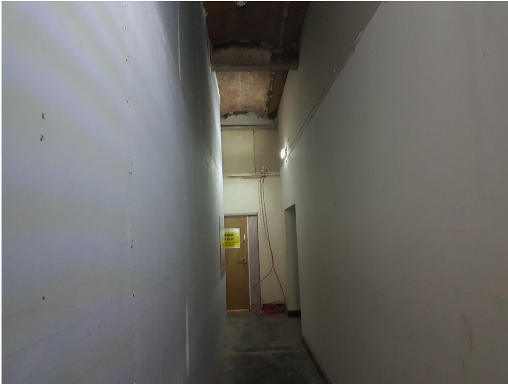
Image 005: Fire Escape Corridor
