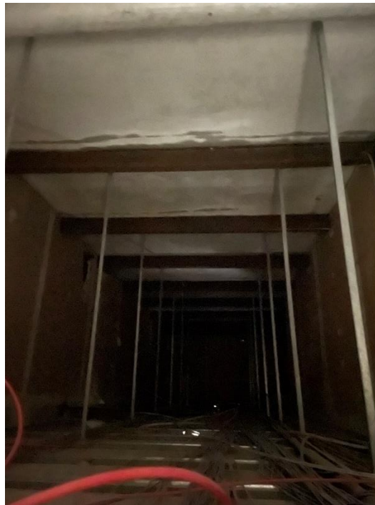
Image 013: Above ground floor suspended ceiling
