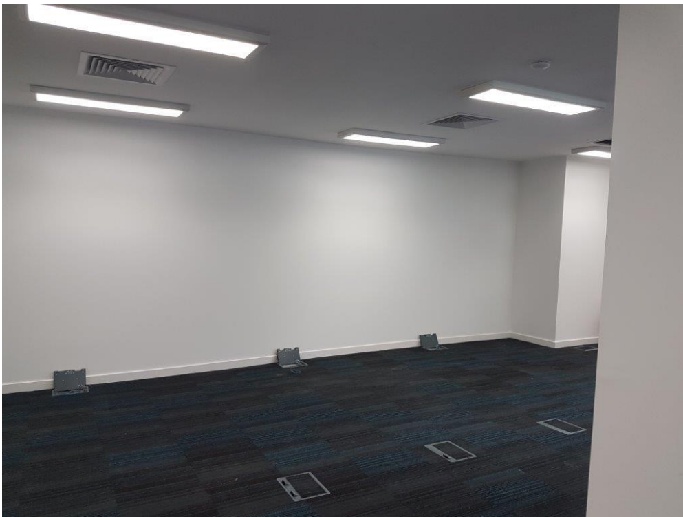
Image 019: Ground floor office typical interior
