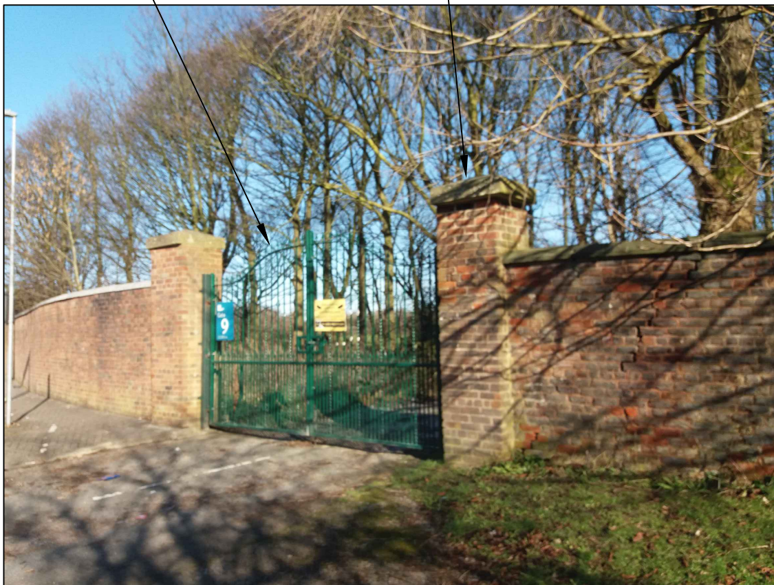
Photo 1: General view of Gate 9 wall.
