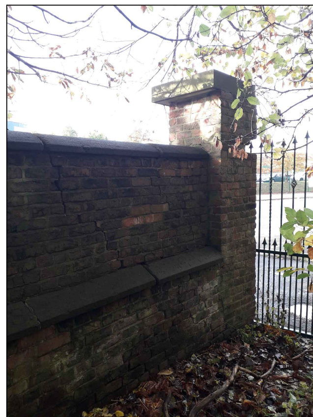
Photo 5: View of internal face of wall.
