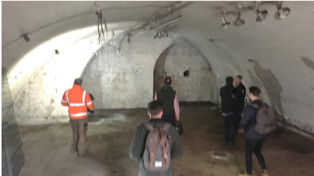
Internal Photos of Arch 3
