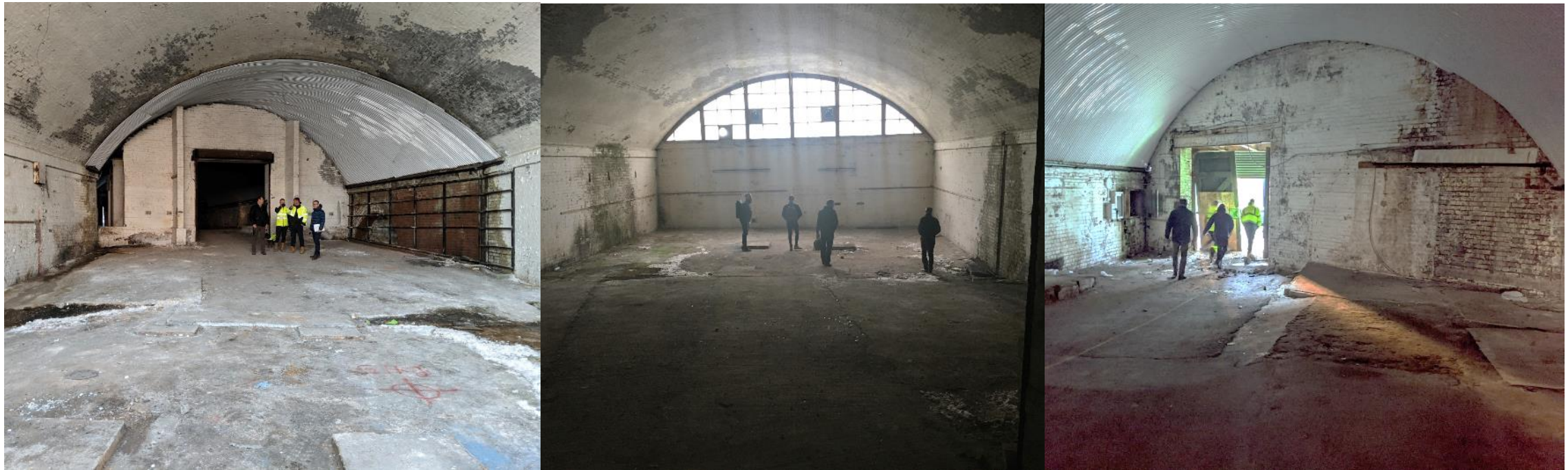
Internal Photos of Arch 10
