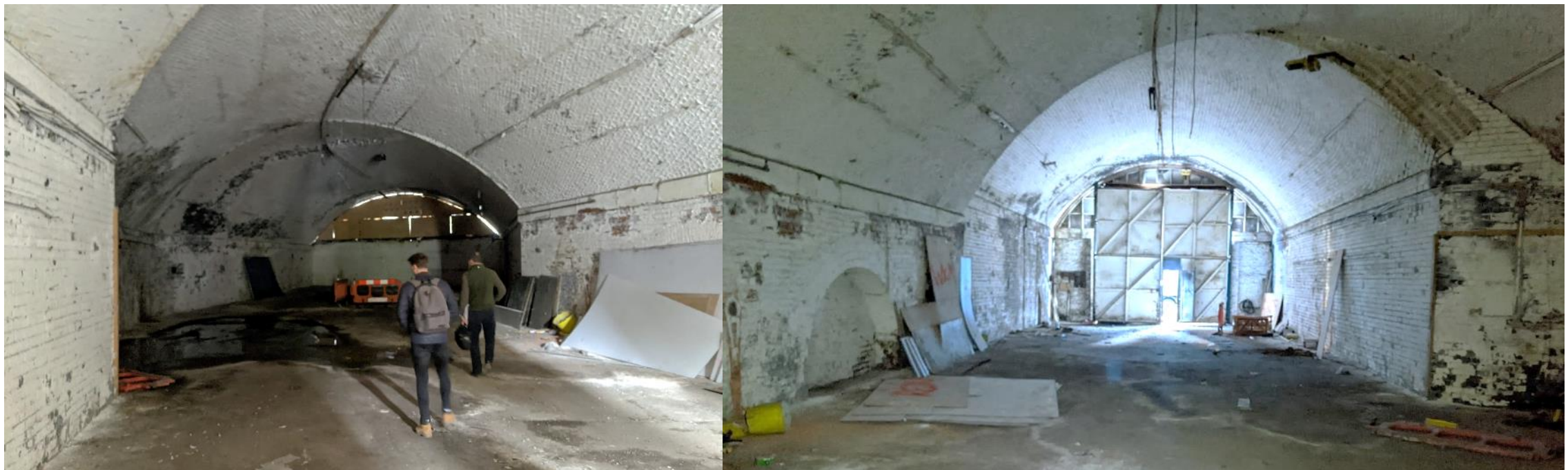
Internal Photos of Arch 11
