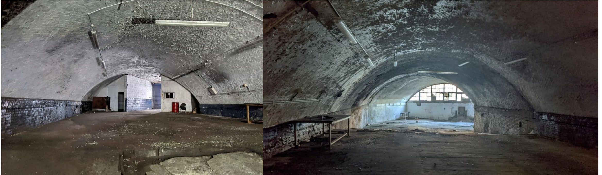
Internal Photos of Arch 8
