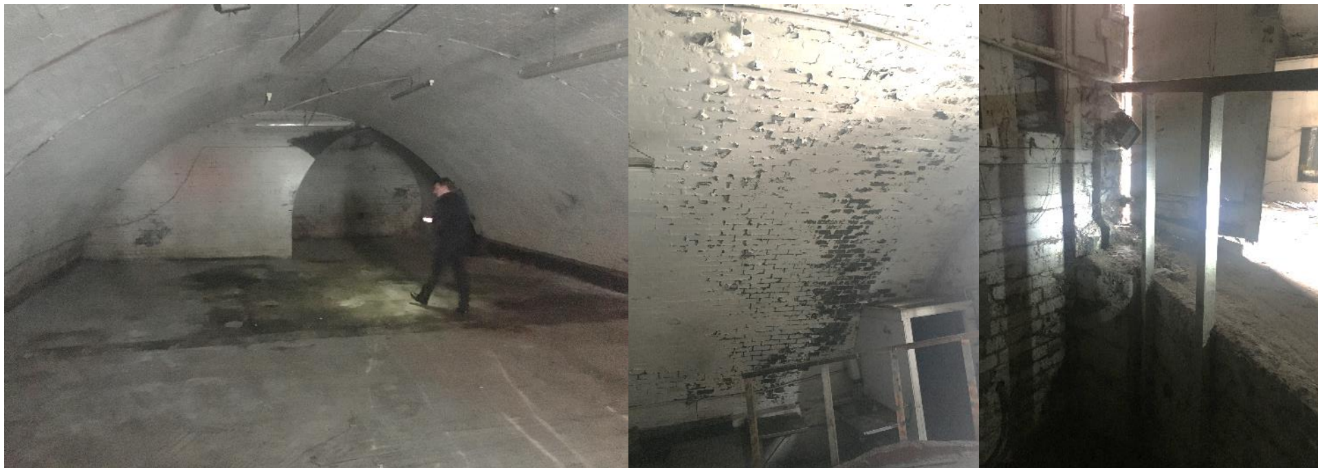
Internal Photos of Arch 4
