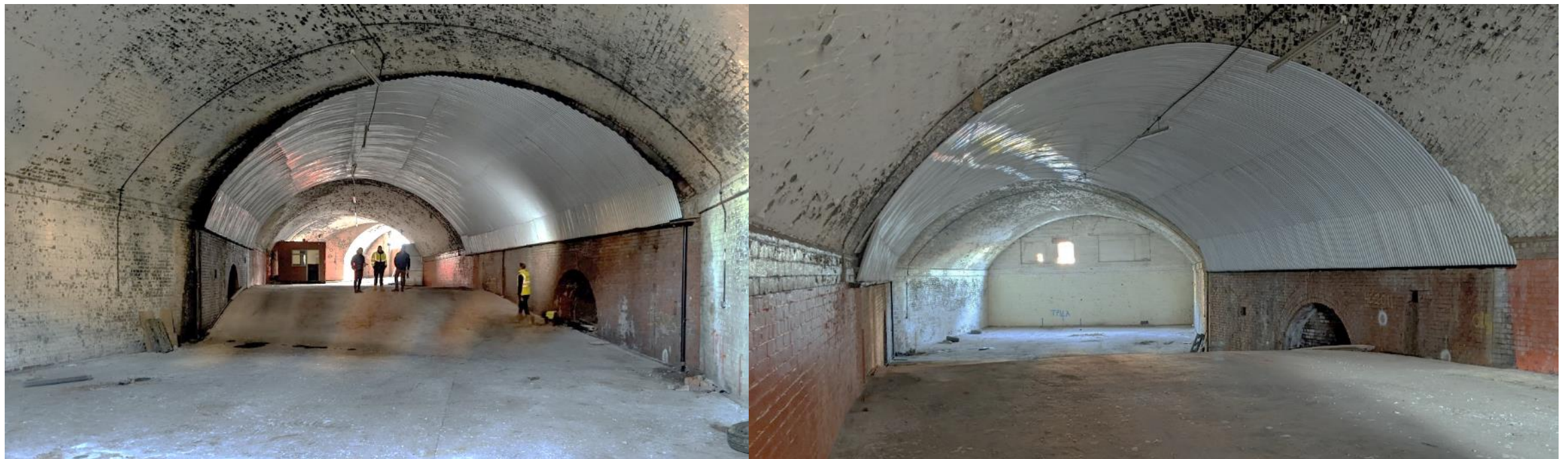
Internal Photos of Arch 9
