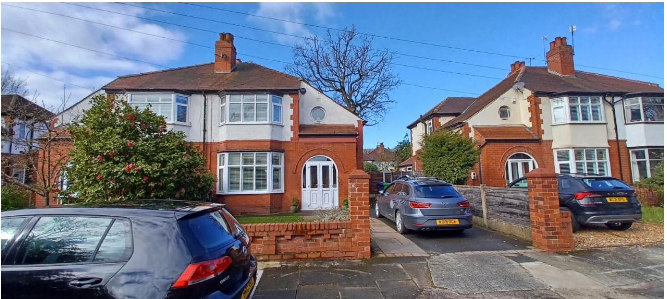
Figure 1. Principal elevation of No.7 Wingate Drive.
