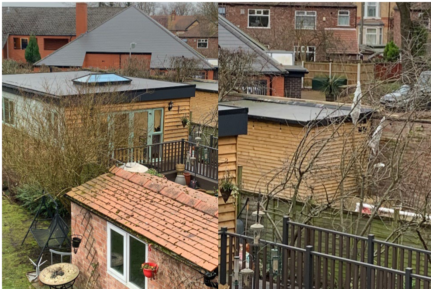
Figure 6. No49 & 51 timber clad out houses.
