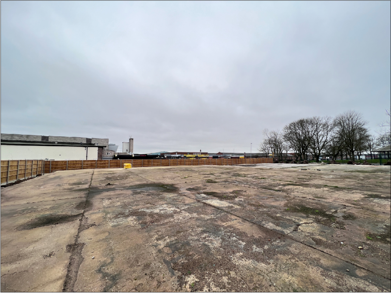
Photo shows that G5 along the south boundary has been removed.
