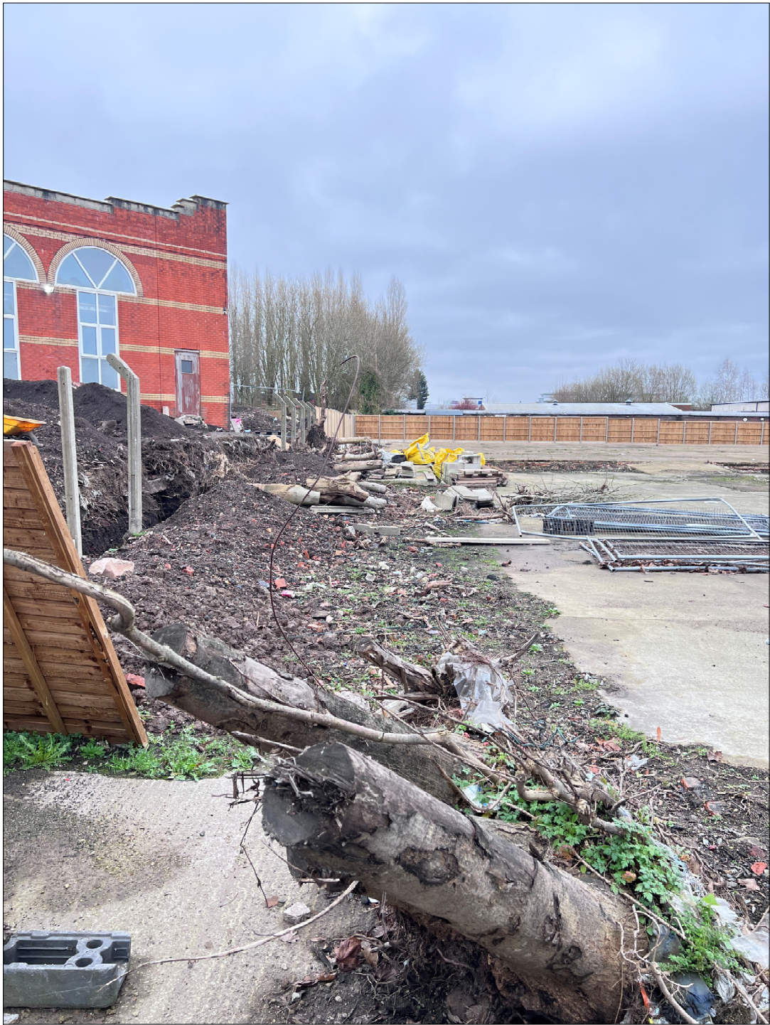
Photo shows that G1 to T3 along the north boundary have been removed
