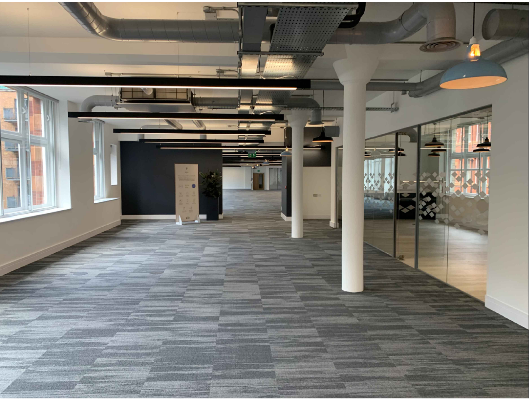
EXISTING PARTITIONS TO BE STRIPPED OUT
