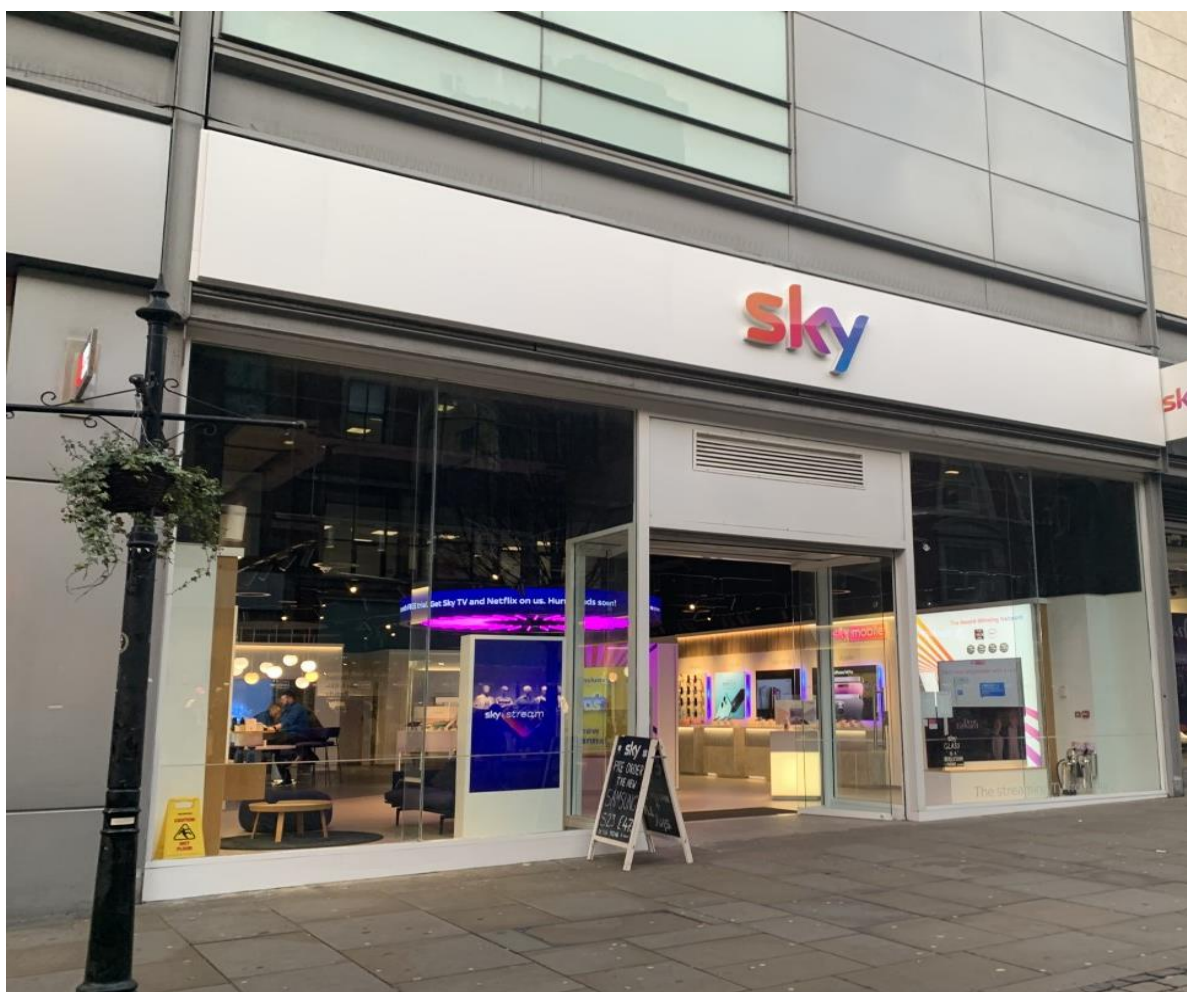
Current unauthorised fascia sign installed and projecting sign installed
