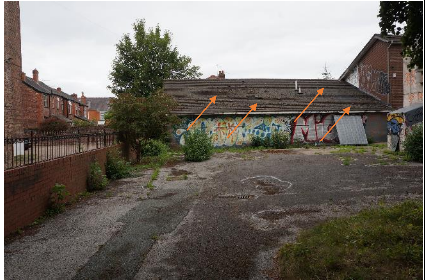
Figure 8: Example locations of broken roof tiles
