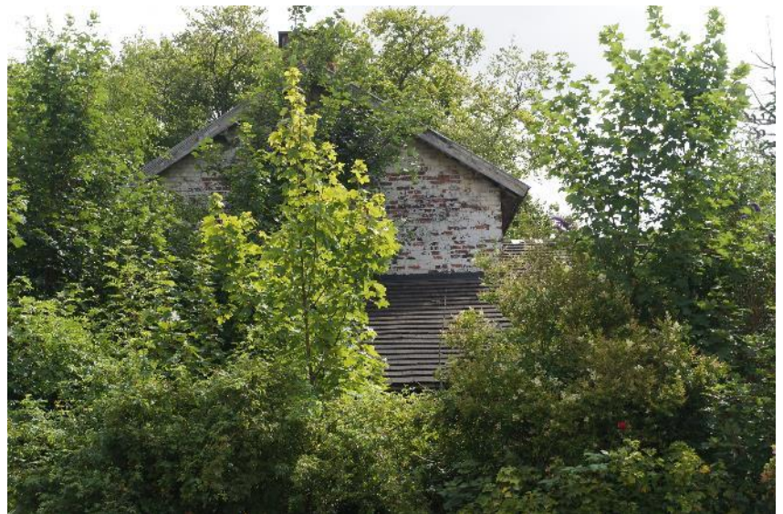
Figure 9: The west gable end of the building obscured by shrubs..
