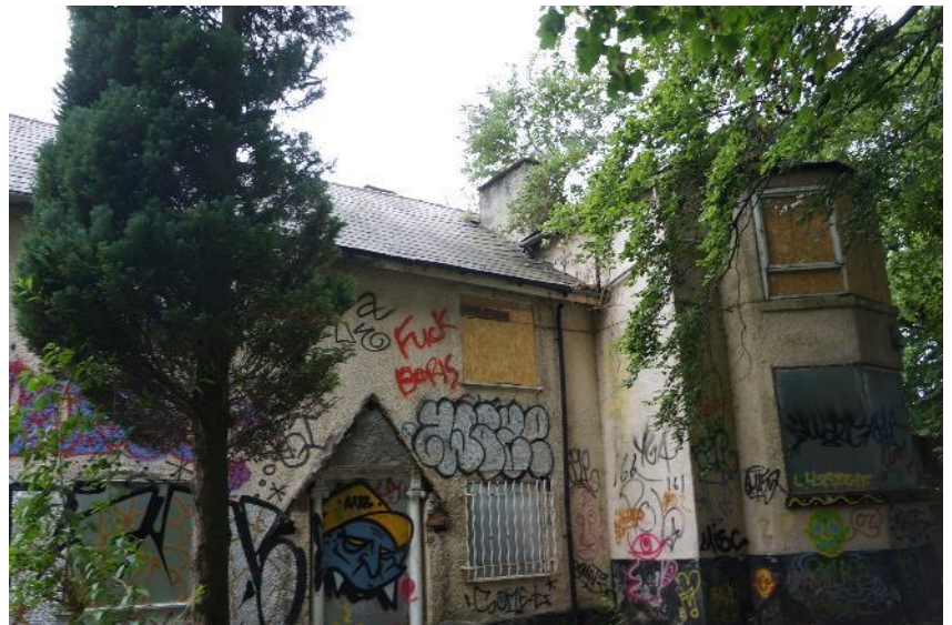
Figure 11: East elevation of original dwelling showing boarded windows.
