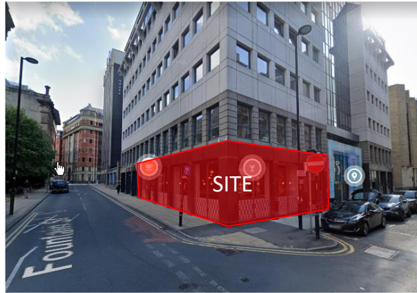
Figure 1 Street view of site
