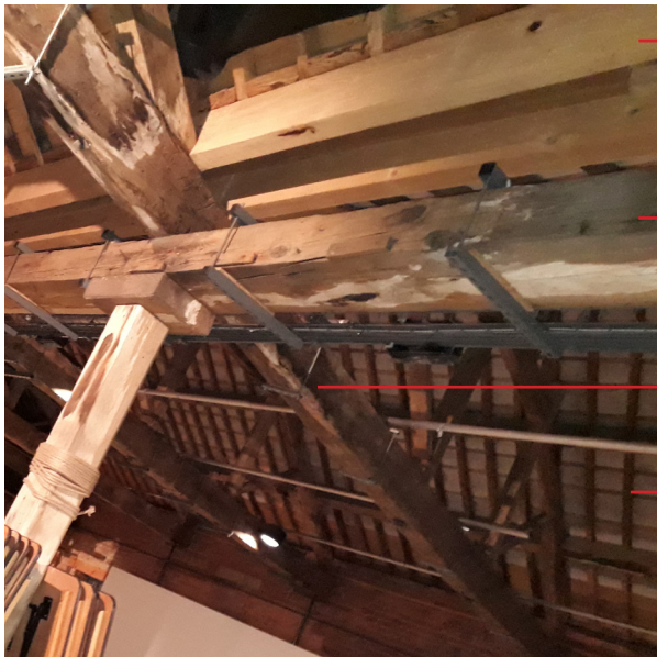
View of a valley beam gutter from below
