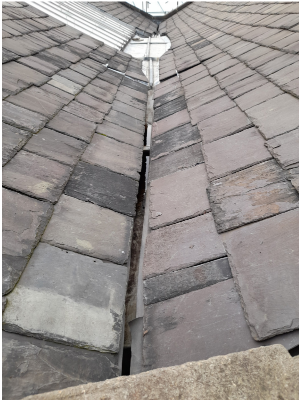
View of a valley gutter from above
