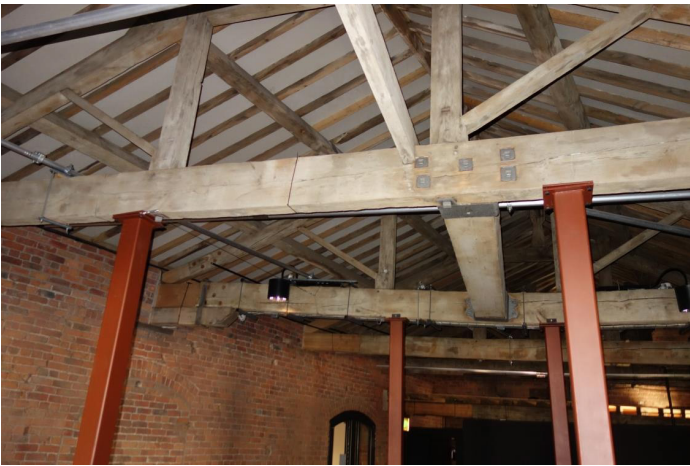
Square Hollow Section columns (4No), serve to prop failed trusses at the East side of Bay 2.
