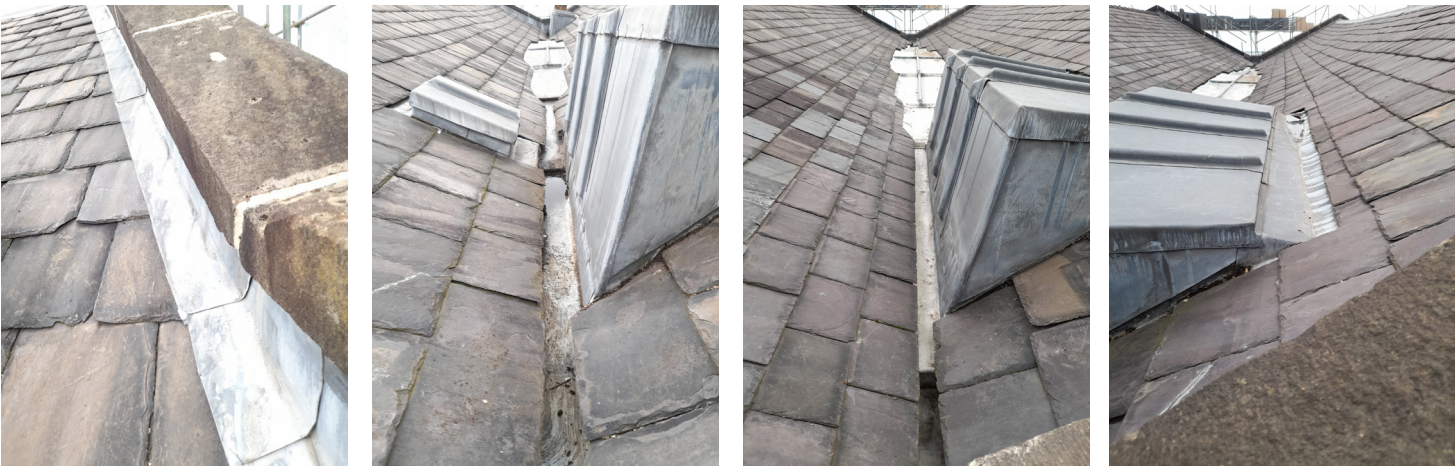
Example images of the existing roof above the Bay 4 Torching. The archive drawings indicate that second hand slates were laid in the 1990’s when the existing torching was installed.
