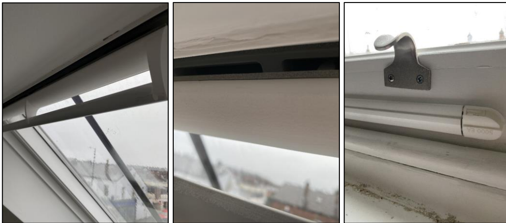
Figure 4.1 - Photographs showing new window trickle vents
