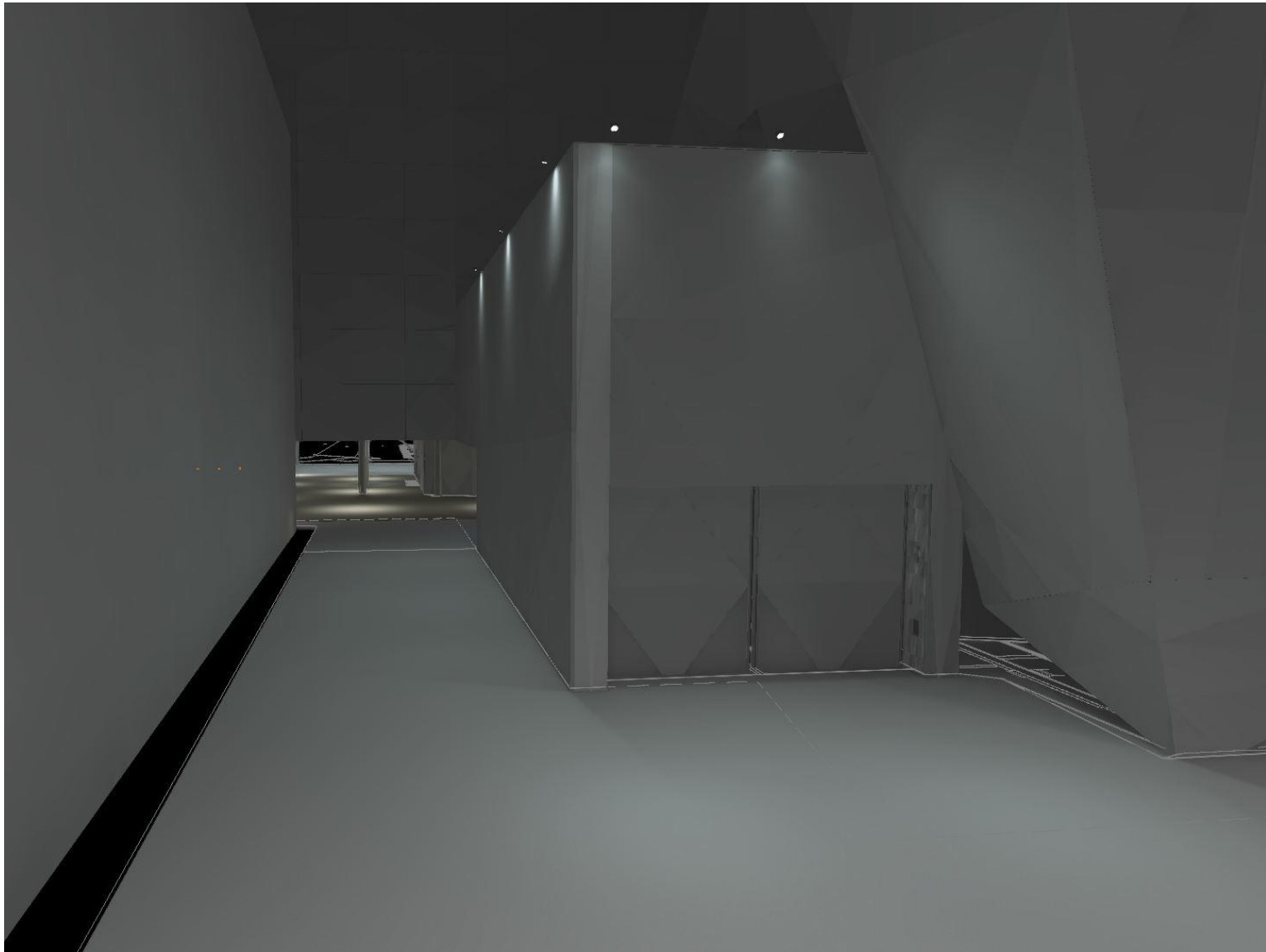
Truck lift parapet lighting ('L2' & 'L3')
