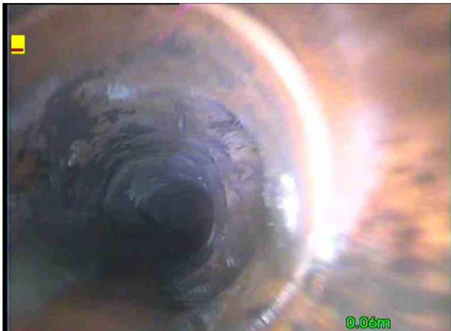
, 00:00:00, 0.00 m Start node type, manhole, reference number: Manhole 3
