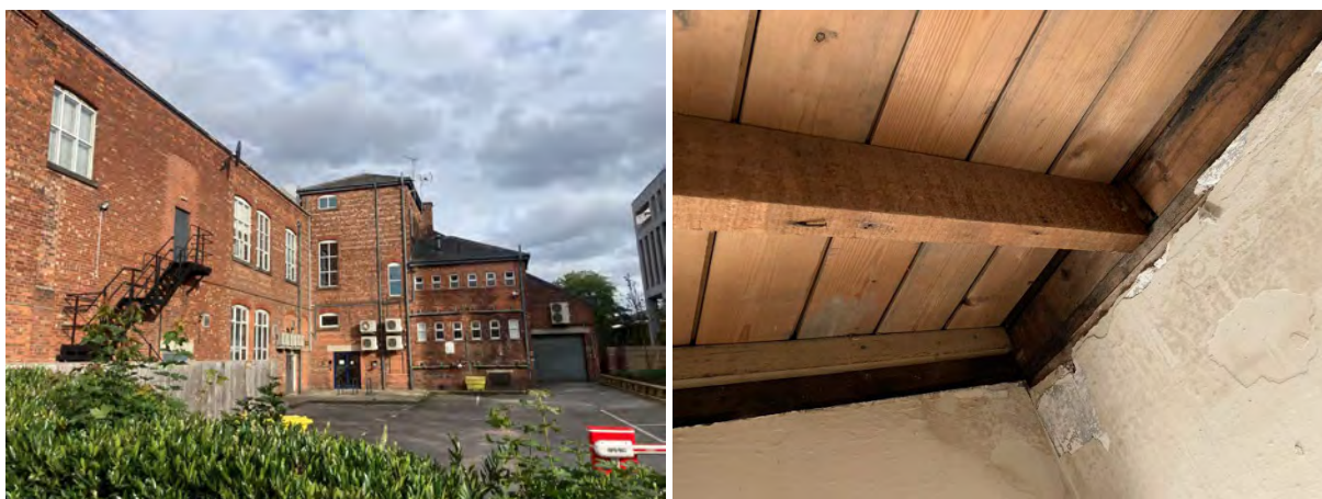
Photograph 5: a) Western aspect of Building 2. b) Exposed roof structure within Building 2.
