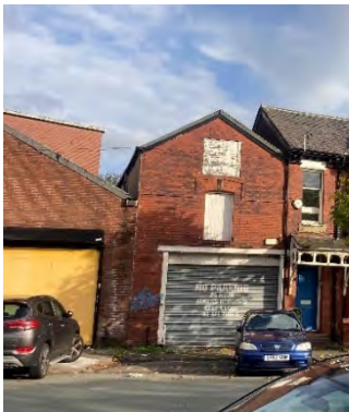
Photograph 9: a) Western aspect of Building 5. b) Damaged roofing felt at apex. c) Crevice present above roller shutter door.
