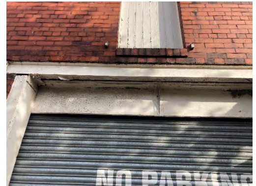
Photograph 9: a) Western aspect of Building 5. b) Damaged roofing felt at apex. c) Crevice present above roller shutter door.
