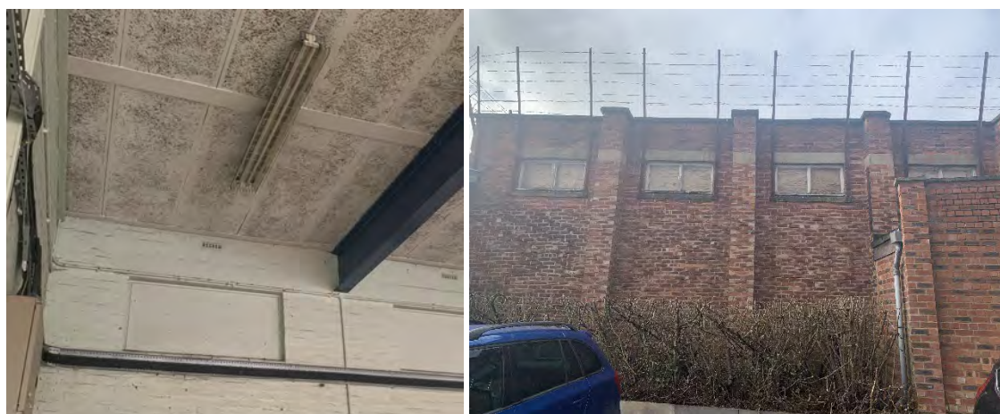
Photograph 10: a) Internal of B06. b) brickwork and crevices on western aspect of B06
