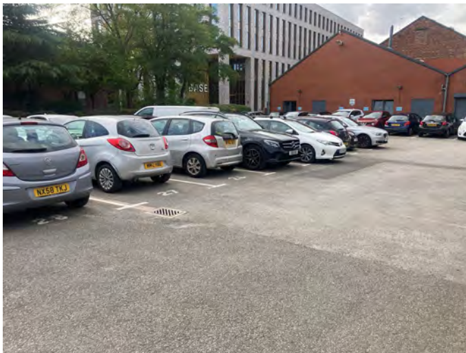
Photograph 1: Hardstanding in the east of the site.
