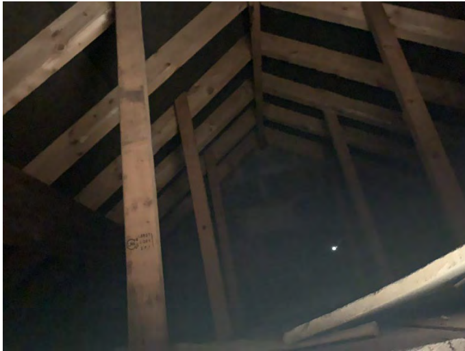
Photograph 8: Roof void within the southern terrace of Building 4
