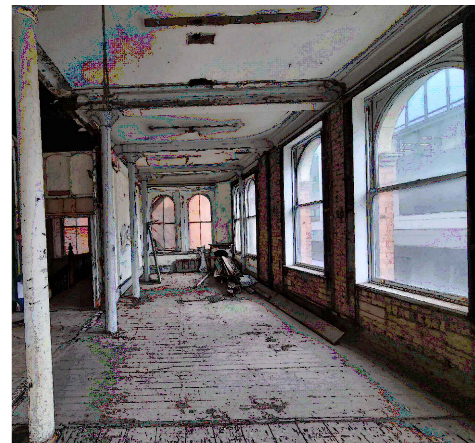
Existing internal window condition ( ref-First Floor )
